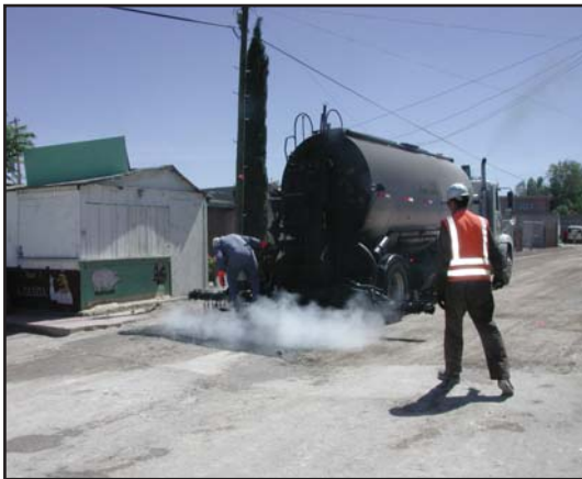
Street paving with an asphalt and crumb rubber mix, Ciudad Juarez
