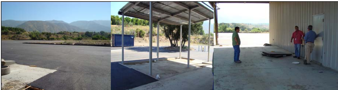
Left: green waste and composting area; Middle & Right: hazardous waste storage areas; Pala Band of Mission Indians, Pala, CA
