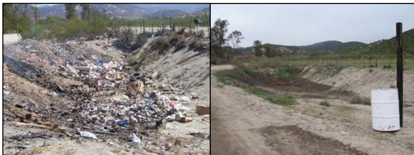
Left: before trash removal in wash; Right: after trash removal in wash; a 200 liter can gives the community a place to put trash; San Antonio Necua Kumiai Community, Baja California, Mexico.
