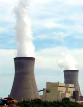
The Rockport Power Plant in Rockport, Indiana, burns coal to produce electricity.
