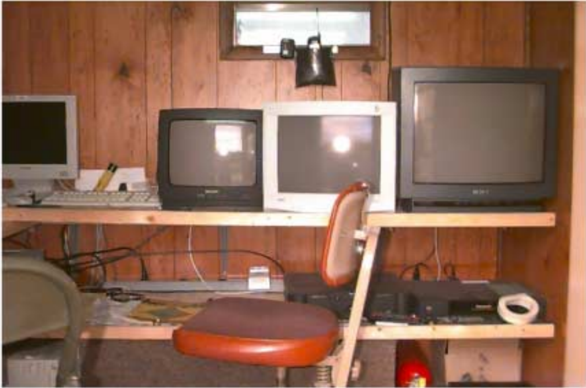
Photo F-5. Port Side of Operator Compartment Showing Picture Displays and Receiver Shelf
