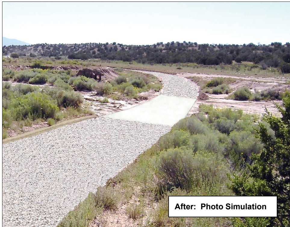
Figure 15. Visual simulation of proposed Buckman Road improvements showing gravel surface and road dip channel crossing.
