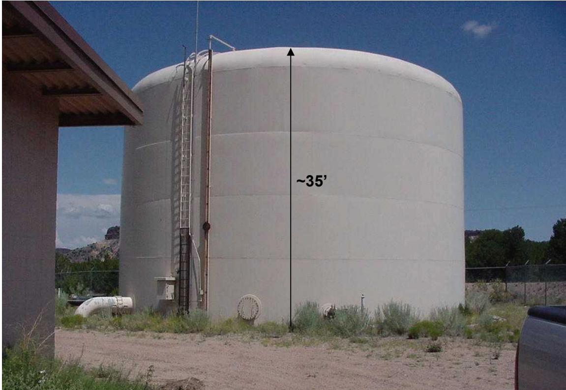
Figure 9. Photograph of existing steel water tank at Booster Station 1.
