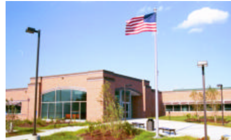
EPA's New England Regional Laboratory in Chelmsford, Massachusetts, is LEED Gold certified.
