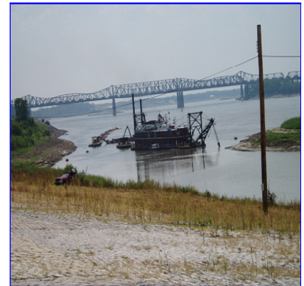
Dredging activities on Mississippi River looking downstream near Mud Island
