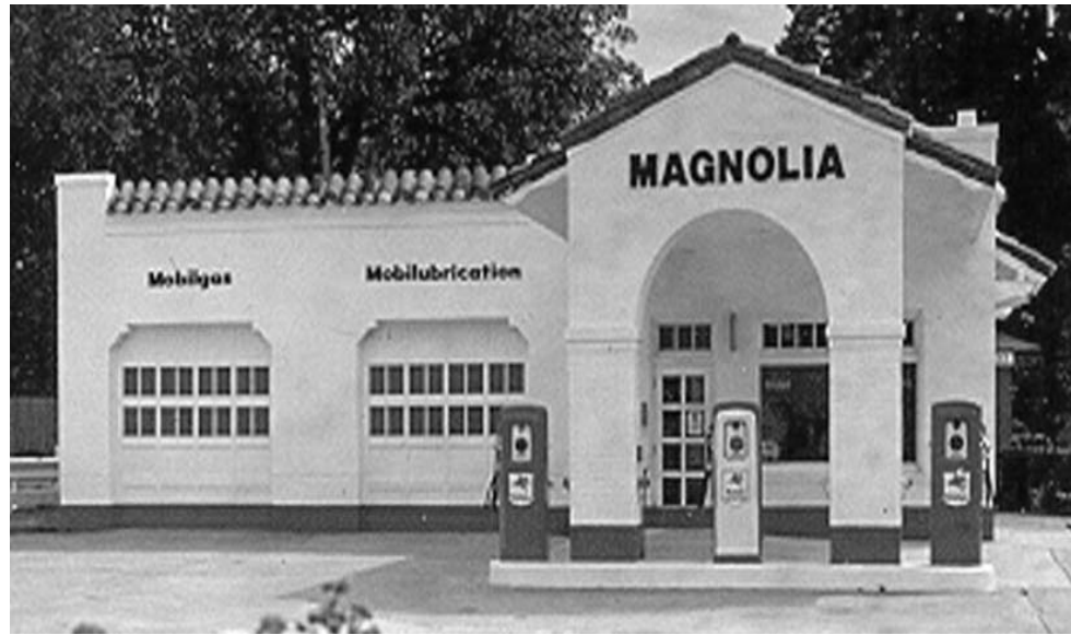
Magnolia Mobil Gas Station, site of the Little Rock Central High School National Historic Site Visitor Center.
