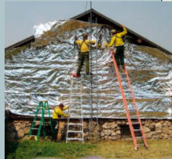
Fire fighters placed protective cover on the refuge manager’s house, which is located on Red Rock Lakes NWR, MT. A lightning-caused fire that started on nearby private land in August 2003 spread onto the pristine wilderness refuge, benefiting wildlife in many ways. (USFWS)
