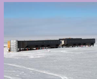
The exterior of the newly completed Amundsen-Scott South Pole Station. Antarctica is the coldest, highest, driest, and windiest of the continents—and the least hospitable to human life. The South Pole Station provides shelter and lab facilities to researchers, including up to 48 who overwinter during the dark austral winter, with an additional 104 berths for summer researchers. Credit: National Science Foundation
