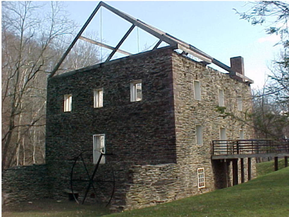
View showing Blackrock Mill looking northeast.
