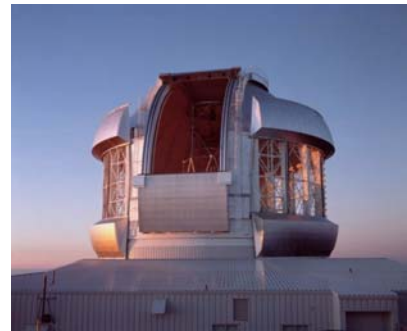
Gemini North dome/enclosure with setting sun (to left) lighting up bottom half of telescope through thermal vents (fully open). The observing slit is partially open revealing the truss and top end of the telescope. Credit: Neelon Crawford, Polar Fine Art; Gemini Observatory/AURA and NSF
