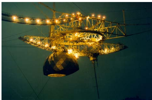
The gregorian dome and its suspension structure over the main deflector of the Arecibo radio telescope, at night. Credit: Arecibo Observatory/NSF
