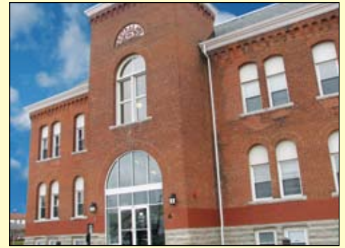
Central School Apartments, once a former school building, now contains 35 affordable apartments for senior citizens. The project involved both certified historic renovation to preserve the only pre-1900 structure in Anderson and new construction. Quality Housing Development, Inc. used a $200,000 AHP grant awarded to Irwin Union Bank and Trust to help complete the project.
