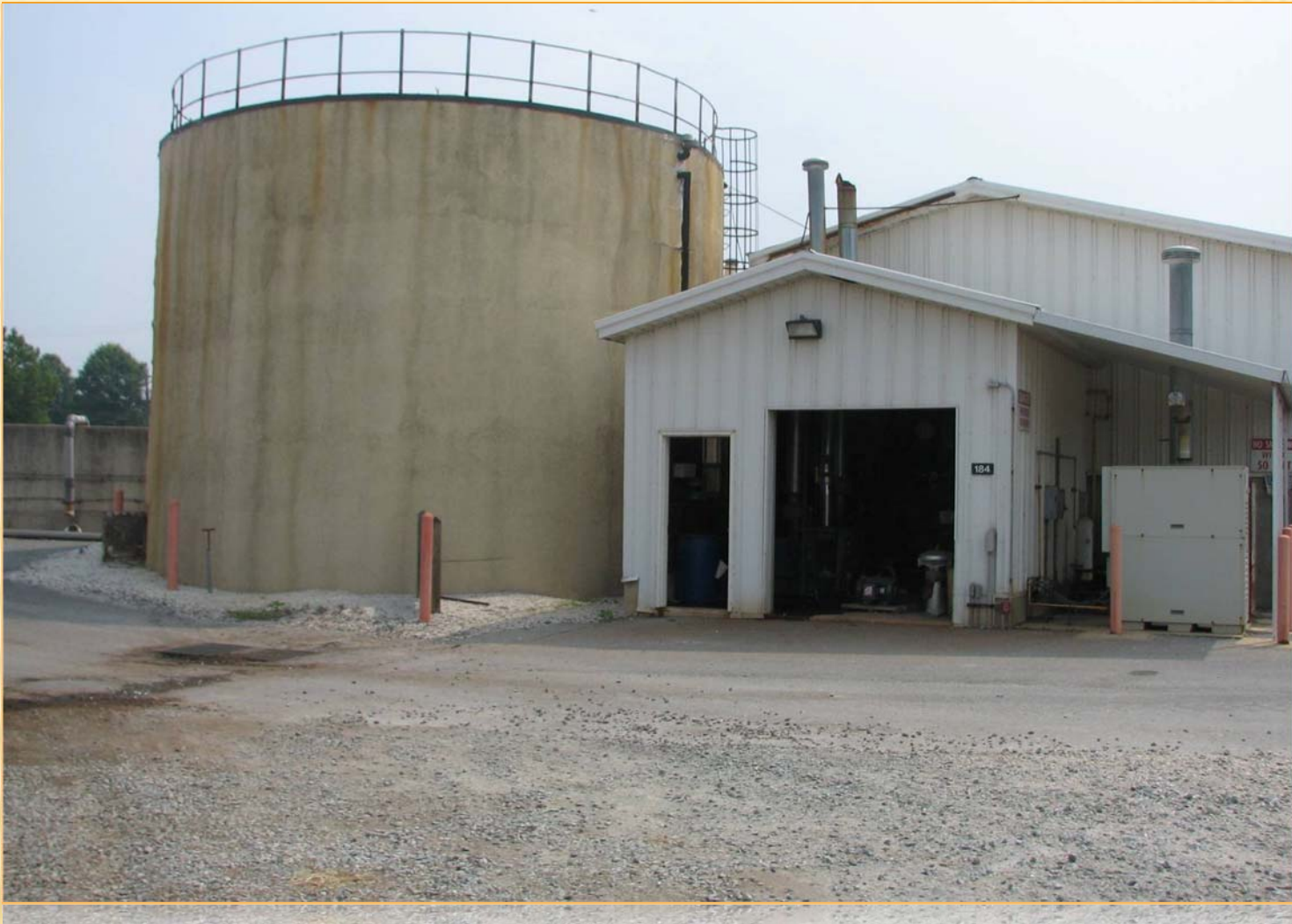
DIGESTER AND CONTROL BUILDING
