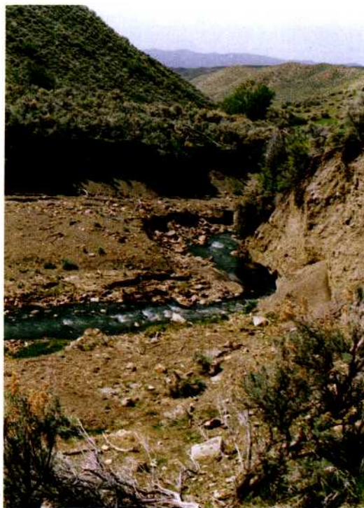
Vertically unstable stream channel.
