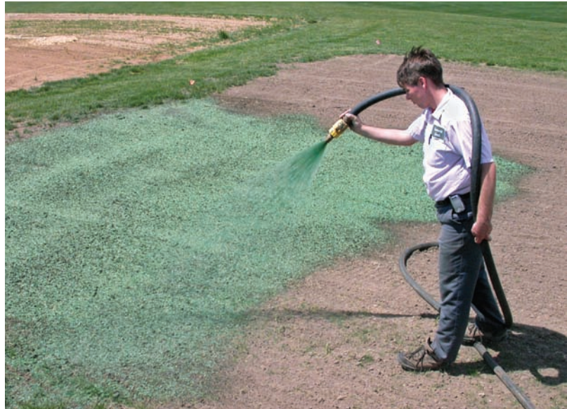
Summit Seed, Inc., employee Dan Pralle sprays a test plot with one of the cotton-based hydromulches developed during the research study on value-added processing of cotton gin byproducts.
