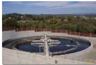
Waste Water Treatment Plants
