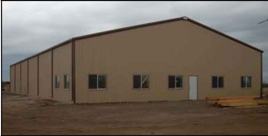
Figure 2-8. Typical Wind Energy Facility O&M Building.
