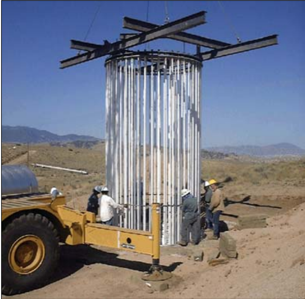
Figure 2-4. Pier Foundation Installation.
