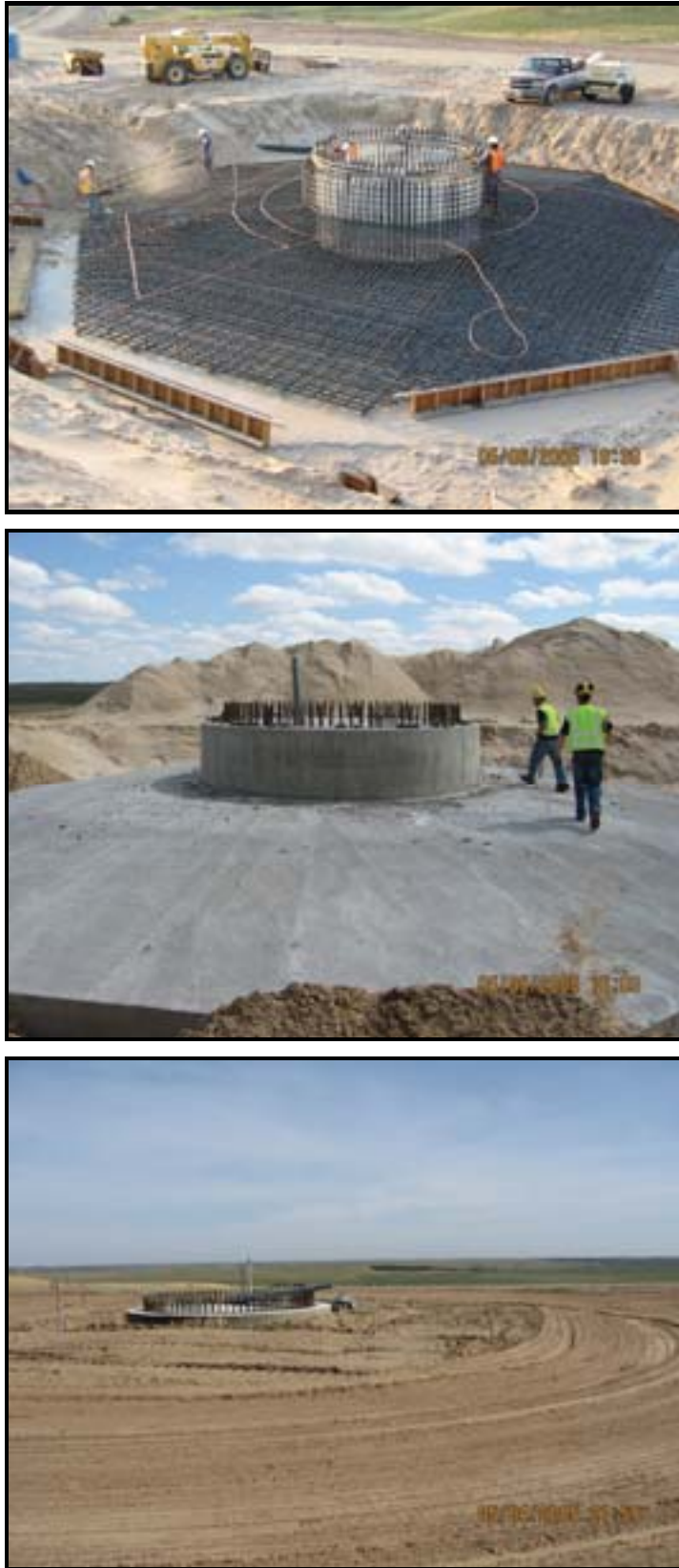
Figure 2-3. Mat Foundation Installation.
