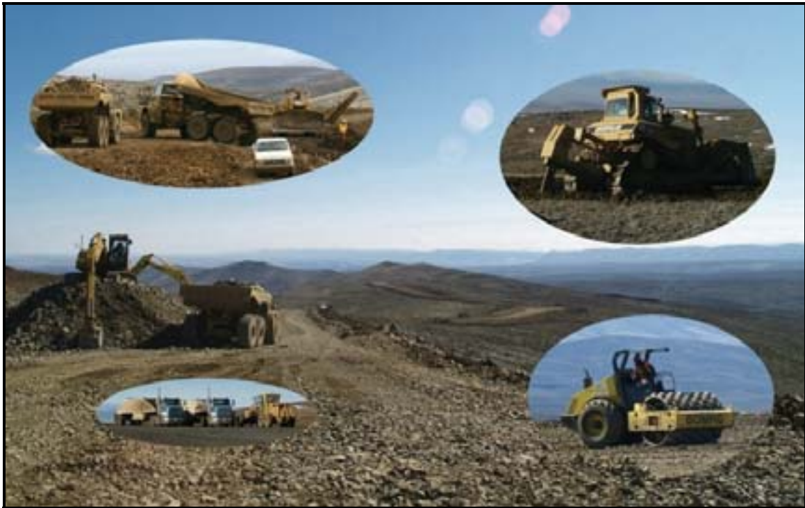
Figure 2-1. Turbine Access Road Under Construction.
