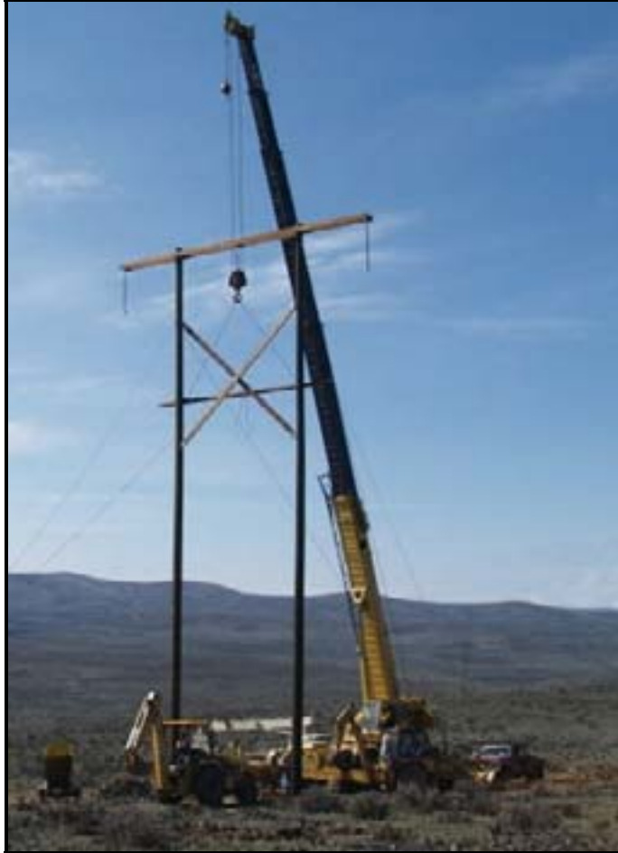
Figure 2-7. Transmission Line Under Construction.
