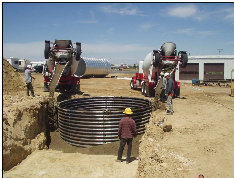
Figure 3-3. Pier Foundation Installation.
