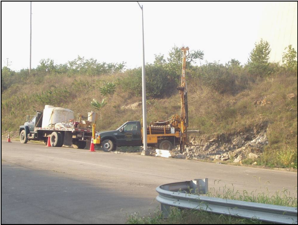
Figure 3-9. Typical Coring Truck and Support Vehicle.
