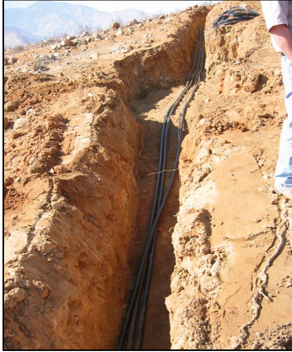
Figure 3-11. Open Trench Example.
