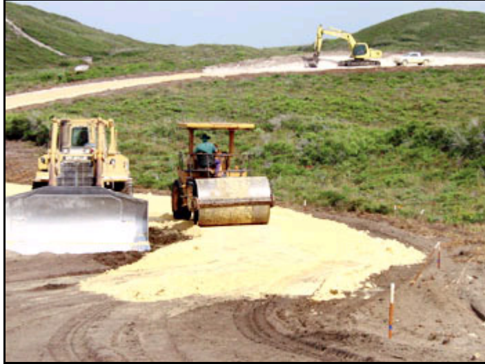
Figure 3-1. Turbine Access Road Under Construction.
