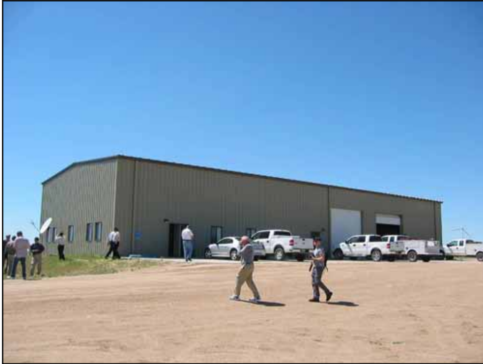
Figure 3-7. Typical Wind Energy Facility O&M Building.
