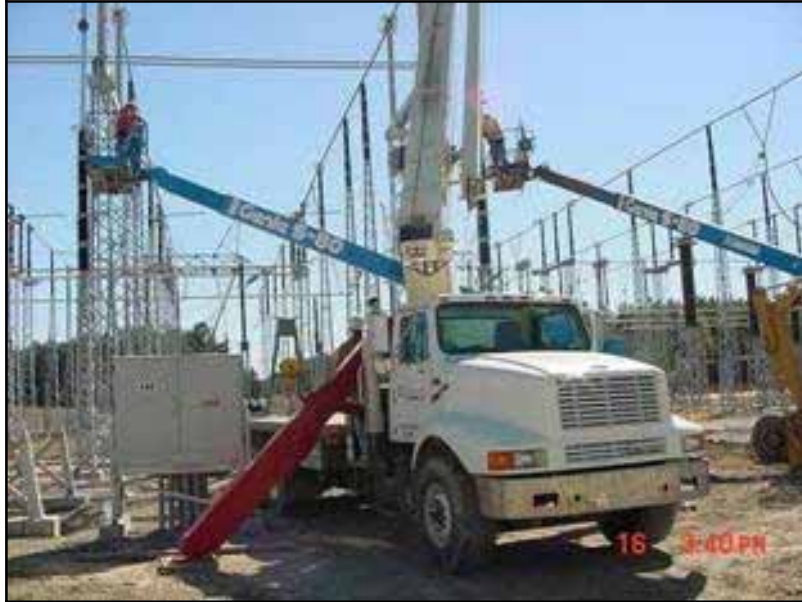
Figure 3-13. Substation Buswork Construction.
