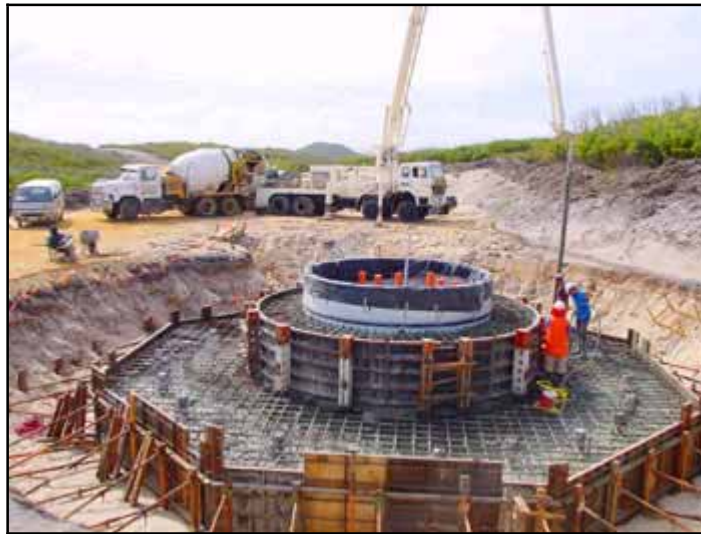
Figure 3-2. Mat Foundation Installation.
