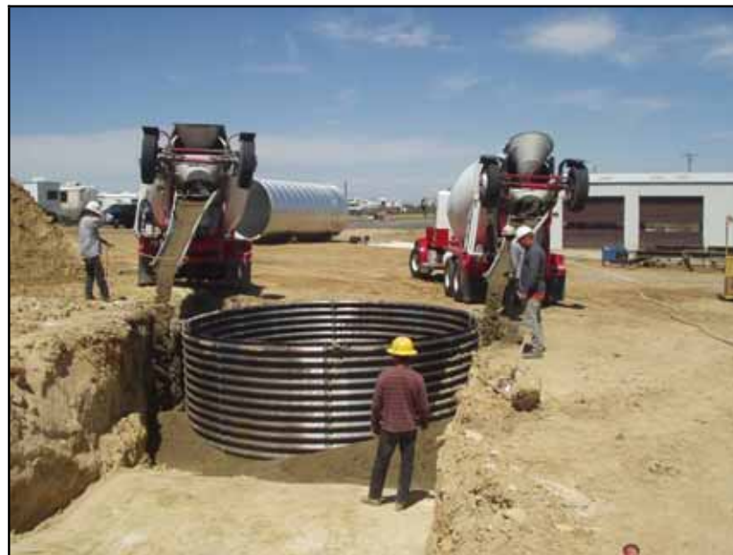
Figure 3-3. Pier Foundation Installation.
