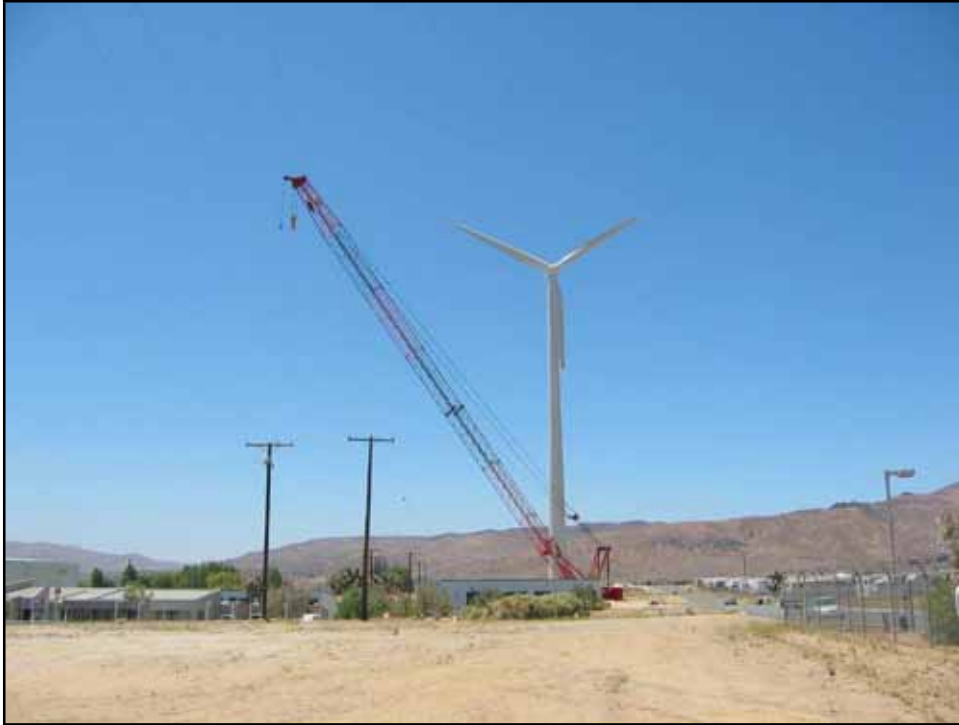
Figure 3-4. Wind Turbine and Crane.
