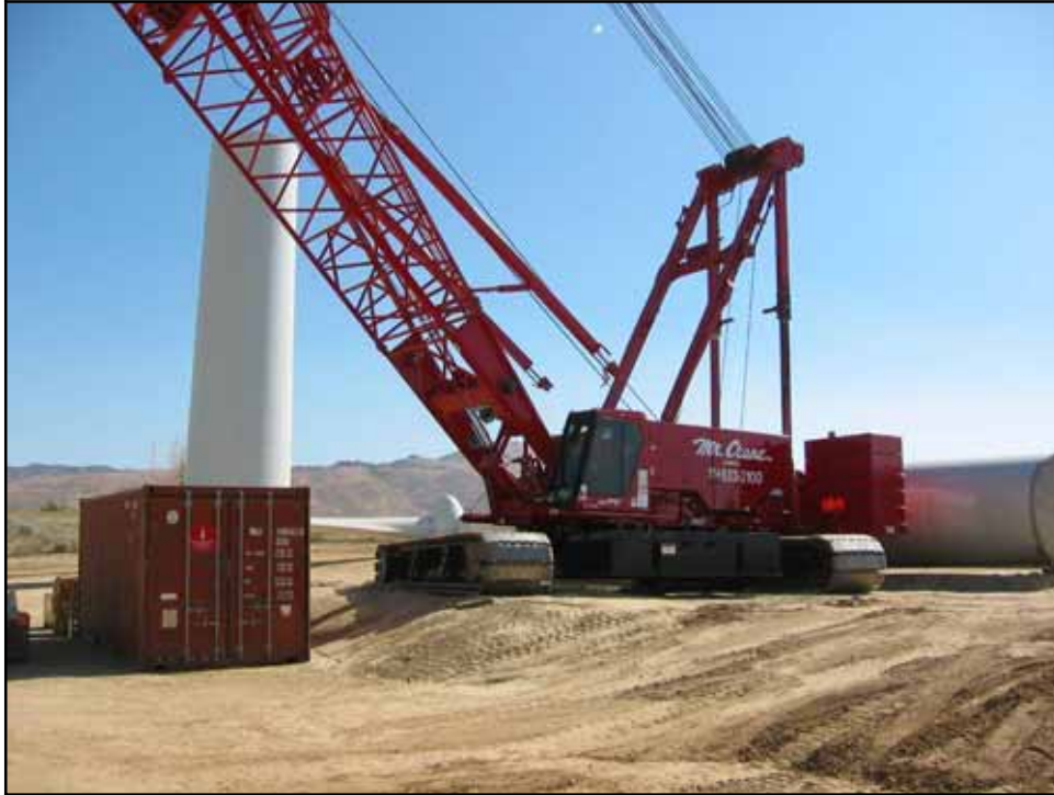
Figure 3-17. Tracked Crane on Crane Pad.
