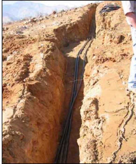
Figure 3-11. Open Trench Example.
