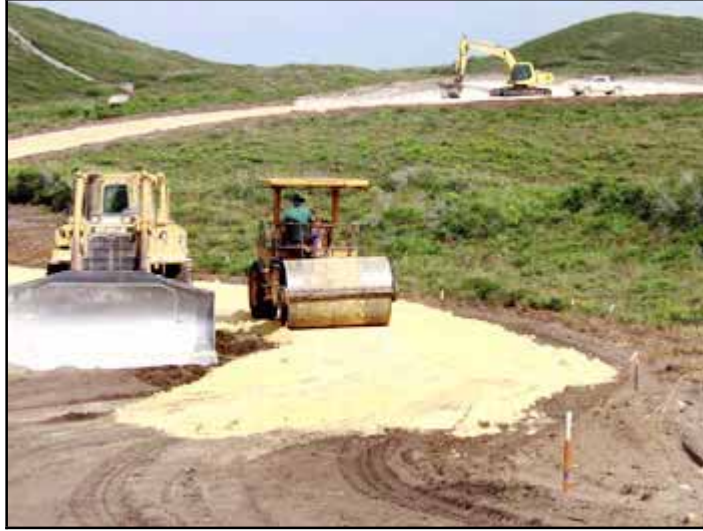
Figure 3-1. Turbine Access Road Under Construction.
