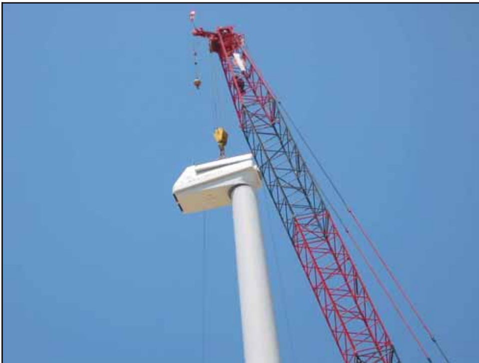
Figure 3-19. Nacelle Placement.
