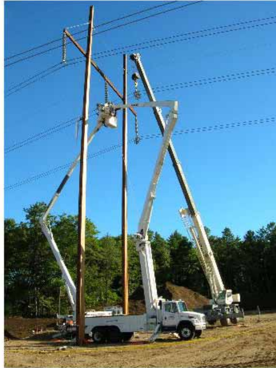
Figure 3-6. Transmission Line Under Construction.
