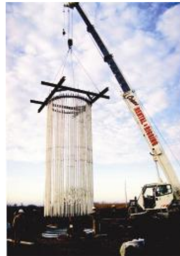
Figure 2.3-10. Bolt Structure for Tower Foundation.
