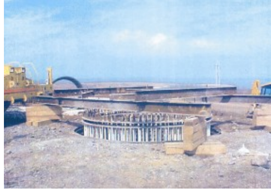
Figure 2.3-11. Foundation Bolts Ready for Concrete Pour.
