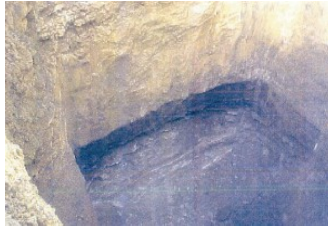
Figure 2.3-8. Excavation of Tower Foundation Hole Following Blasting.
