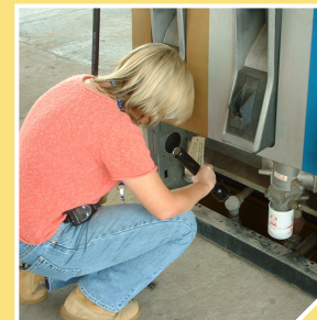
Inspecting under the dispenser
