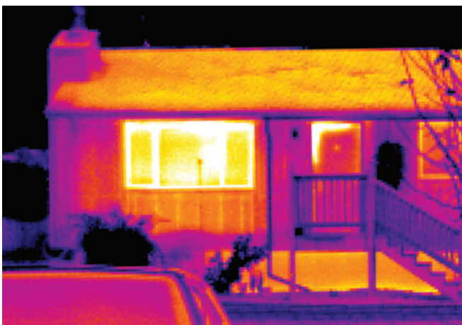
Figure 2. The infrared picture of this house (taken on a cold winter day) shows inadequate roof insulation, an uninsulated basement, a door seal leak and poor wall insulation behind a baseboard heater under the window (see studs).
