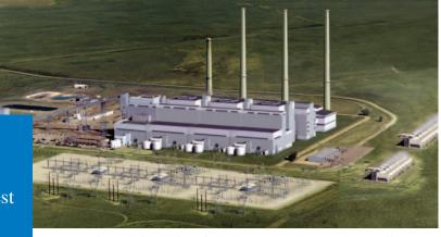
At completion, the Holcomb Station Expansion Project will add three new 700-megawatt generating units to the existing 360-megawatt plant. Tri-State will own two of the new units.
