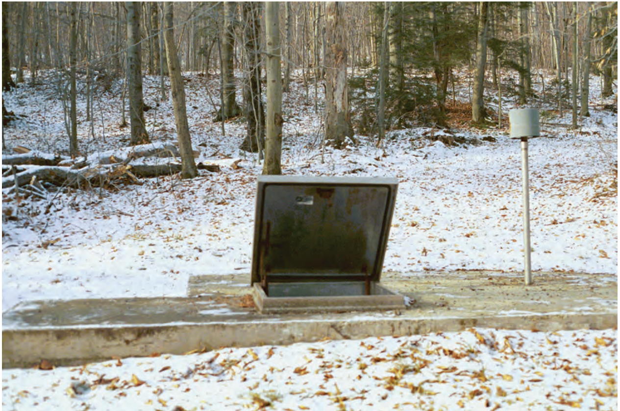
Figure 42. Worthington Fire District Spring 2, westward view, Worthington, Massachusetts.
