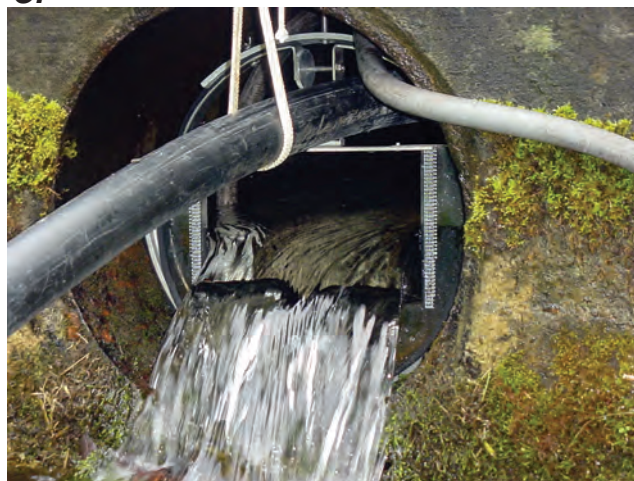
Figure 7. Red Mill Spring in Clarksburg, Massachusetts, showing A , two cisterns at upper center right, storage tank at left, and seepage melting snow at center, southeastward view; B , stage-discharge recording site on northwest side of Route 8, southeastward view; and C , close-up of weir installed in culvert with suspended 2-inch intake pipe for golf-course pump.
