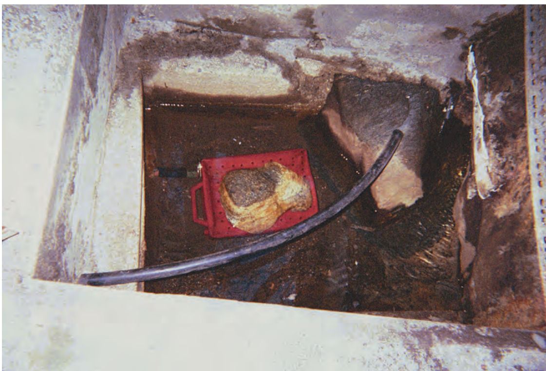
Figure 5. New Belden Tavern Spring in Becket, Massachusetts showing A , covered collection basin against boulder, northwestward view; and B , water flowing into collection basin from under boulder. Photographs by Joseph Cerutti, Massachusetts Department of Environmental Protection.
