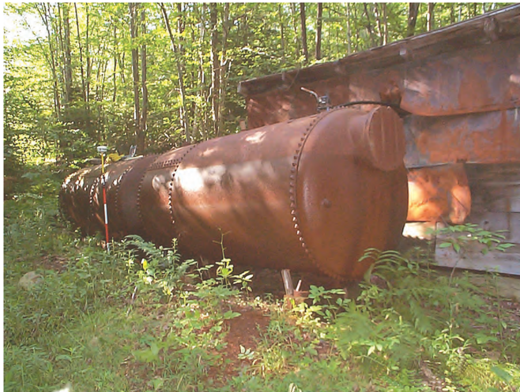
Figure 20. Whitcomb Summit Spring in Florida, Massachusetts, showing A , collection structure, southwestward view; and B , steel collection tanks and pump house, northward view.
