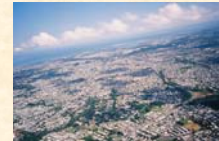
Urban Sprawl: Suburban expansion in the San Juan Metropolitan Area
