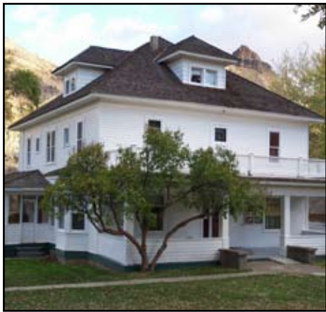
The James Cant Ranch House.
