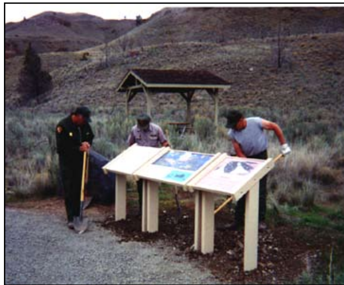
Maintenance staff installs new interpretive waysides.
