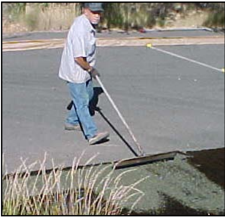
Road crews chipseal the park's parking lots.
