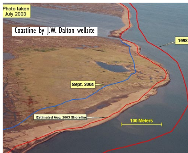
Photographic assessments of erosion along the coastline within the TLSA. The J.W. Dalton test well site is 3 km east of Pitt Point in northcentral TLSA. Cameron Point West is 14 km east of Pitt Point.
