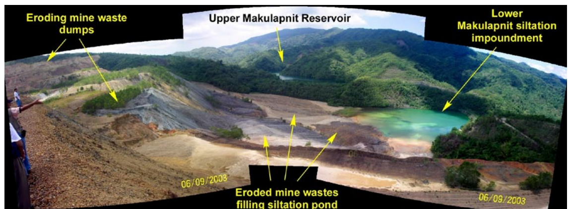
Photographic panorama showing erosion of mine waste dumps into the lower Makulapnit siltation impoundment. Digital composite of three photographs by H. Miller, J. Madsen, taken in June 2003.
