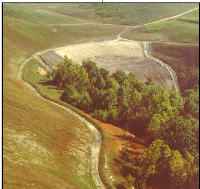
Under the Surface Mining Law excess spoil can be placed in valley fills, under carefully controlled conditions.
