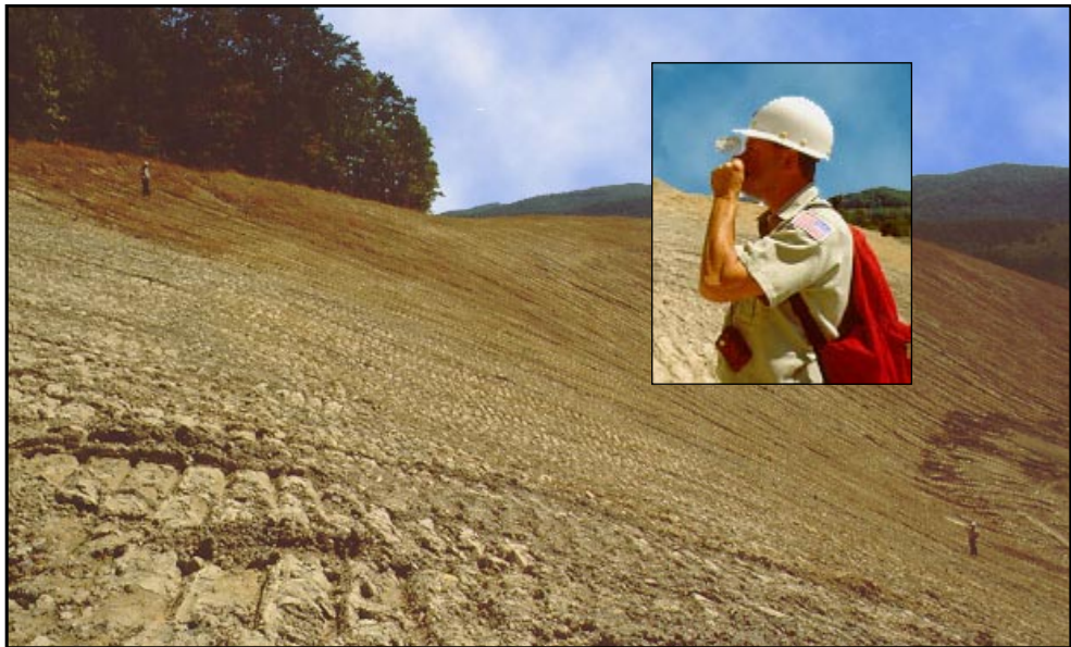
Inspectors check the regraded slope on reclaimed mine land to be sure it is in compliance with the mining and reclamation permit.
