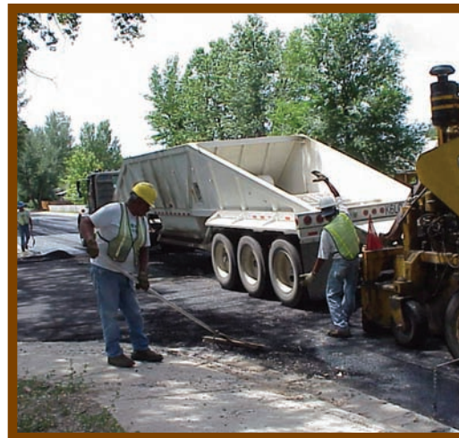
Road construction crew at work repairing street.
