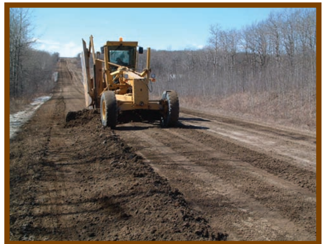
BIA road crew grading dirt road for local access to homes.
