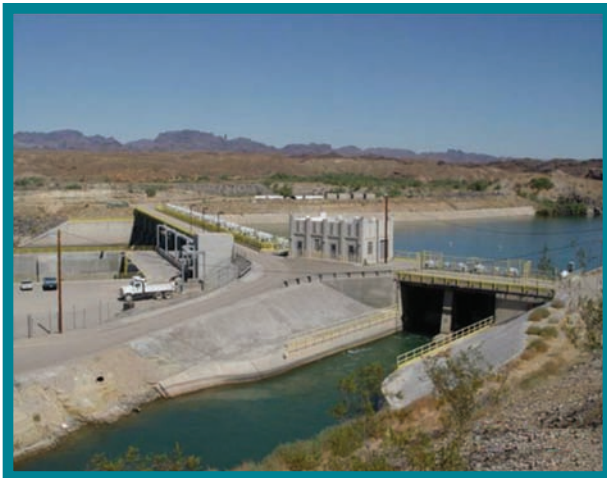
Headgate Rock Dam, Colorado River.
