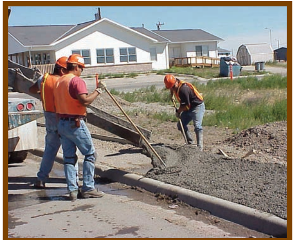
Construction crew pouring concrete sidewalk.
