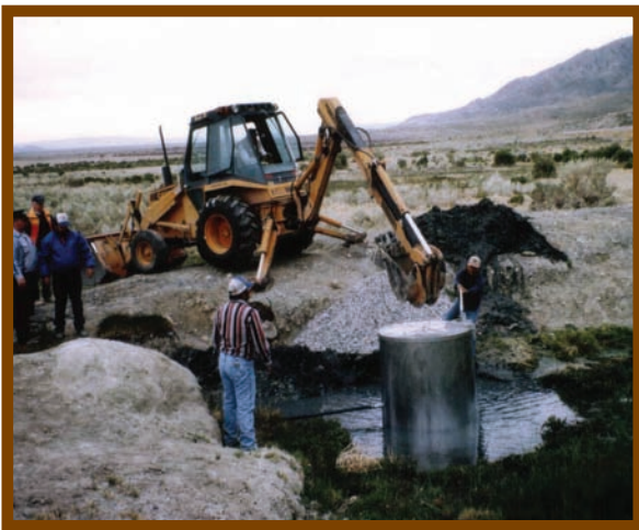
Installing a spring box at Walker River Reservation.
