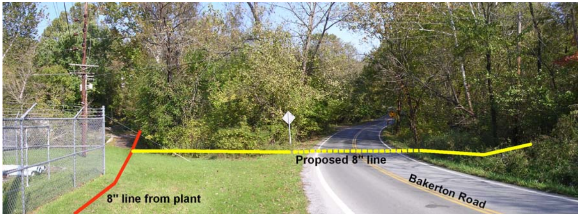
Figure 4: Project area in vicinity of water treatment plant.
