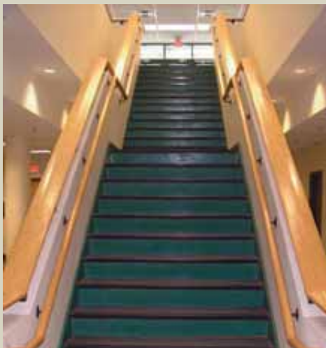
The prominent location of this recycled-rubber staircase encourages walking instead of elevator use.
