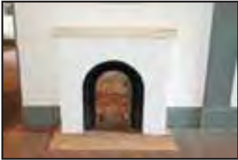
One of two fireplaces remaining with an arched opening. (John Martini, 2005)
