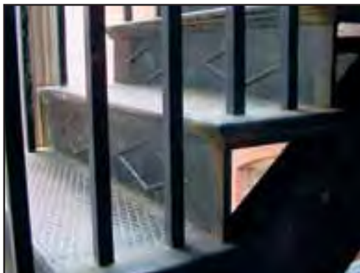
Stair #4 - This cast iron staircase was replicated in 1974 based on the original construction. (Jane Lehman, 2005)
