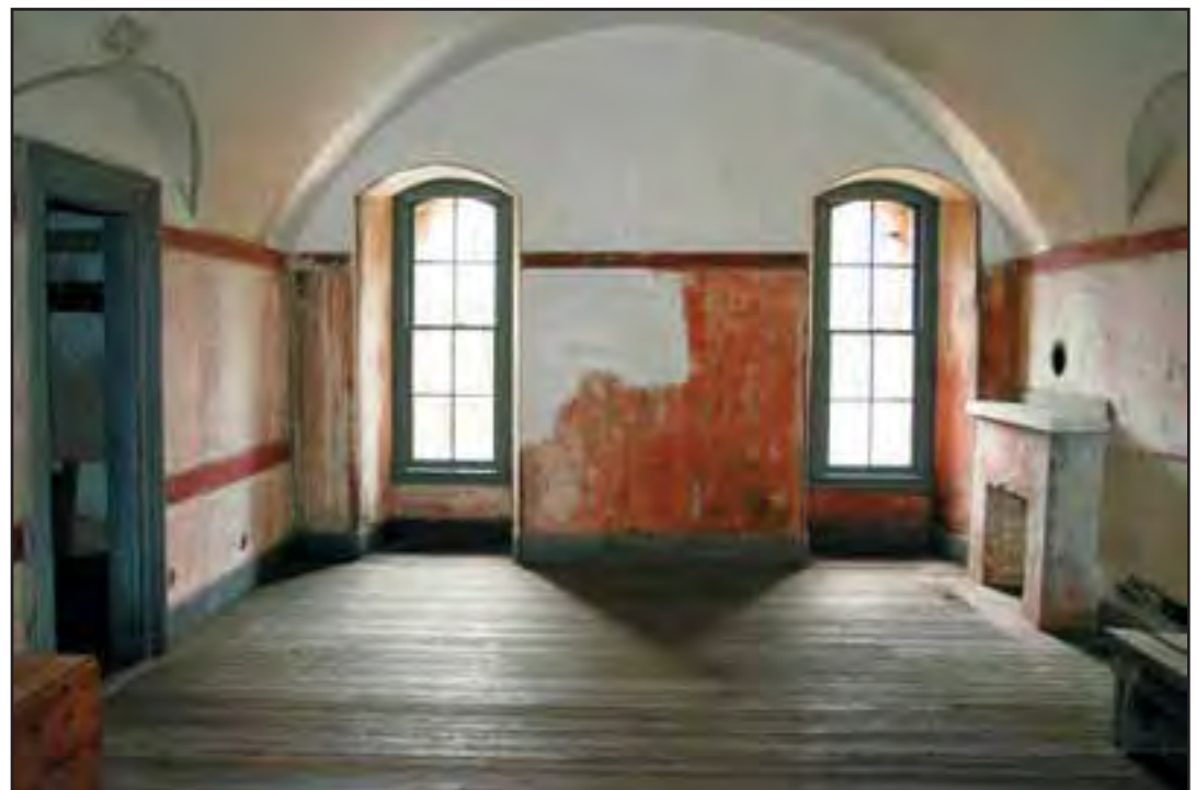
The outline of a previous, original brick wall is visible in the communication arch between enlisted men's quarters 2 & 3. (John Martini, 2005)
