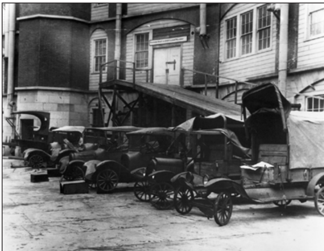
Figure 14. Photograph: Vocational School, viewed from the parade, circa 1924-1925. Credit: Fort Point NHS Collection, Golden Gate National Recreation Area.
