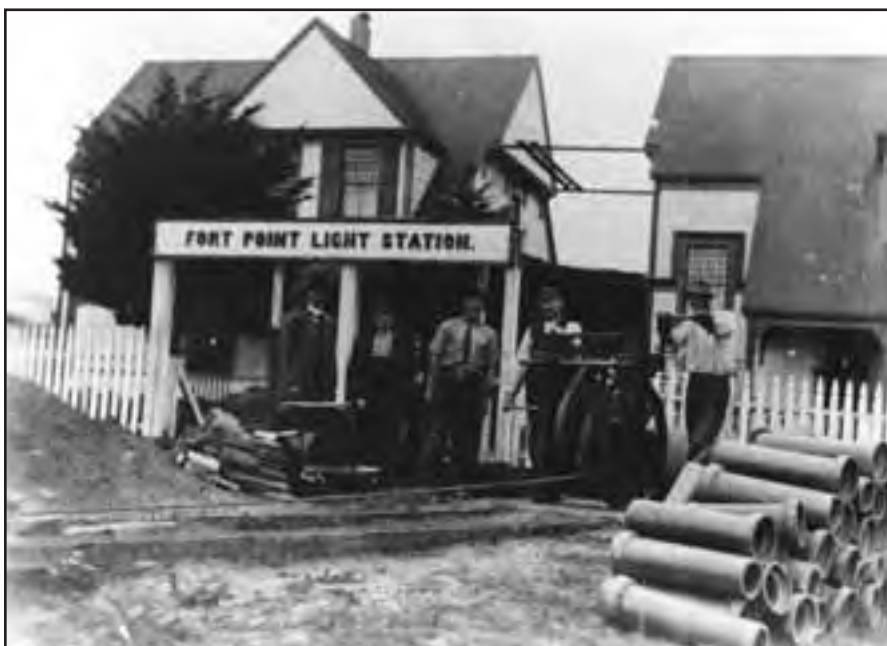
Below: Two of the assistant keepers' houses at the Fort Point Light Station were built atop the hill south of the fort. A windlass helped haul supplies up the steep slope to the "wickies" homes. Terra cotta pipes in the foreground were for plumbing. Photo circa 1910. Credit: Fort Point NHS Collection, Golden Gate National Recreation Area.
