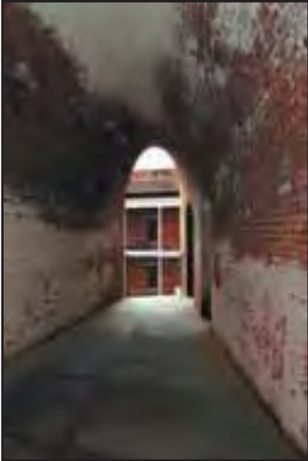
This 3rd tier casemate narrows towards the parade end forming a parabolic arch. (John Martini, 2005)
