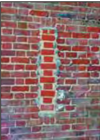
Former rifle slit on south flank filled in with brick. (Jane Lehman, 2005)
