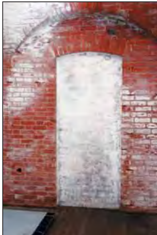
The original doors and brick infill walls are visible in the 3rd tier stores. (John Martini, 2005)
