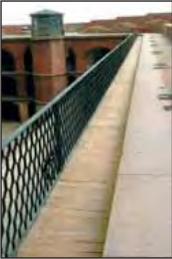
This 3-foot wide walkway and railing above the gallery on the southwest gorge elevation was replaced in a 1973 project. Beyond is the penthouse over stair #3. (John Martini, 2005)
