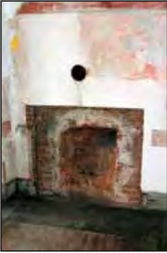
It is apparent from the remnants in this non-commissioned officer's room that the fireplaces were not part of the fort's original construction. (John Martini, 2005)
