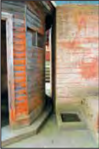
The remnants of the WWII searchlight housing are adjacent to the penthouse for stair #1. (John Martini, 2005)
