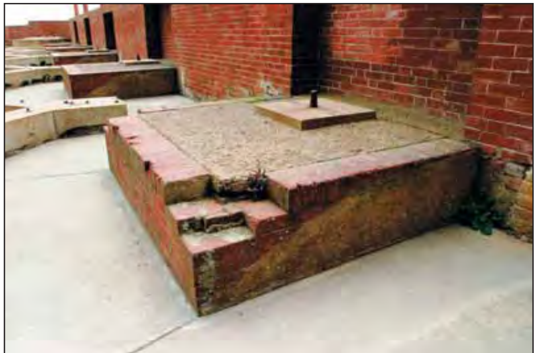
Along the southwest barbette wall is a series of 11 platforms designed to hold 32-pounder guns. (John Martini, 2005)
