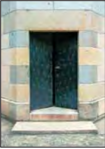
Courtyard level doors into stair #2. This is one of the few pairs of heavy wood doors original to the fort's construction. (John Martini, 2005)
