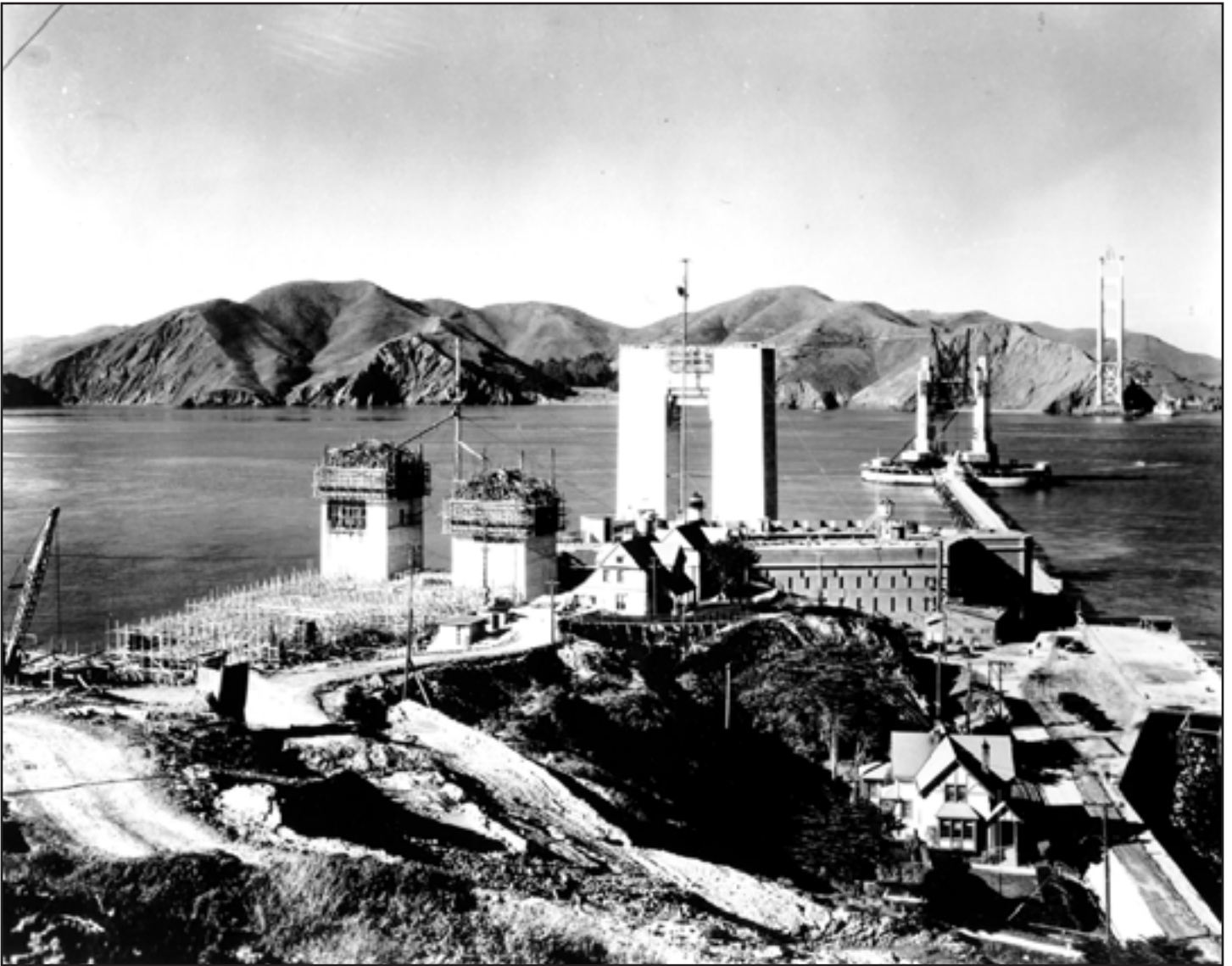
Figure 16. Photograph: Golden Gate Bridge construction, Lighthouse Keeper's Houses, viewed from bluff above Fort, circa 1933. Credit: Fort Point NHS Collection, Golden Gate National Recreation Area.
