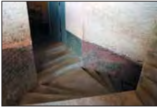
Stair #1 - The steps to the surgeon's room lead from an intermediate landing between the 1st and 2nd tiers. (John Martini, 2005)
