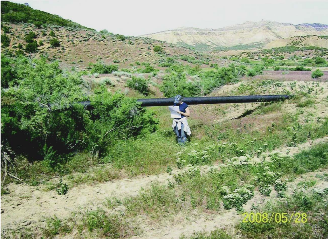
FIGURE 12 – 8" Pipeline Exposure (111+00)
