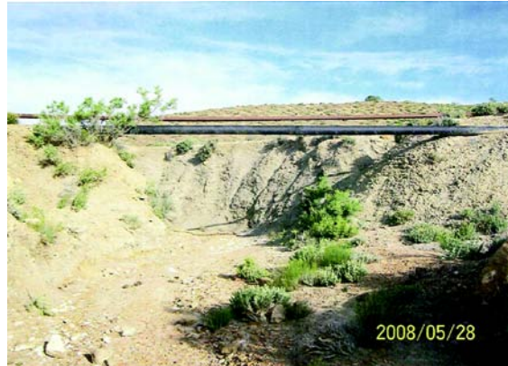
Ephemeral Drainage Crossing (189+45)
