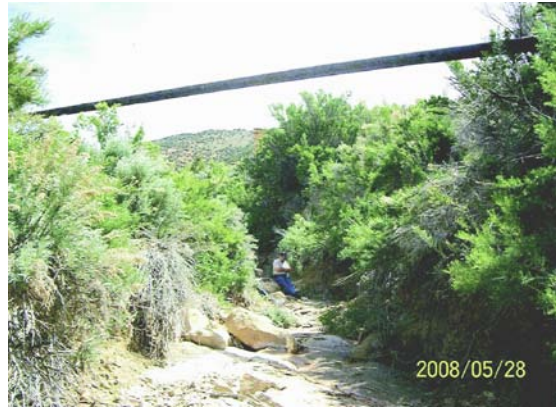
Munger Creek Crossing (29+78)
