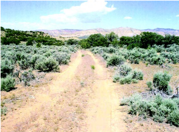
Road Conditions at 30+00
