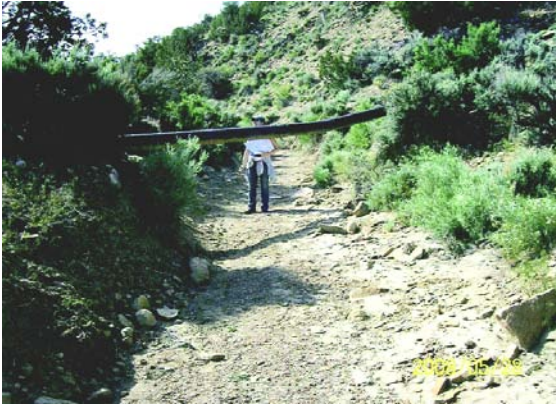
Ephemeral Drainage Crossing (140+25)
