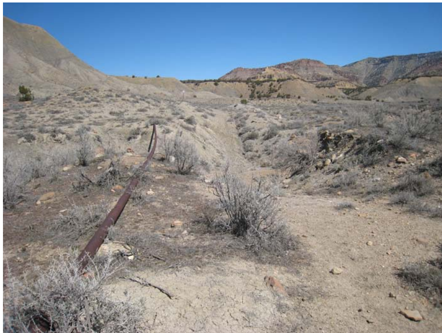
Figure 3-10: Exposure of Existing 8-Inch Pipeline
