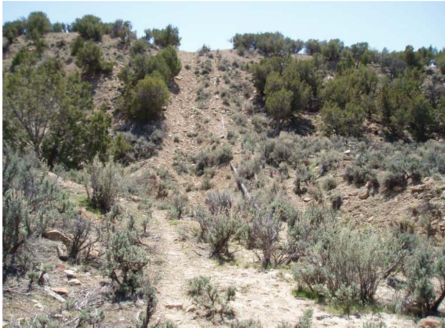
Figure 3-9: Existing 8-inch Pipeline Exposure and Disturbed Area
