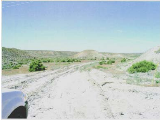
Garmesa Access Road from Valve Set
