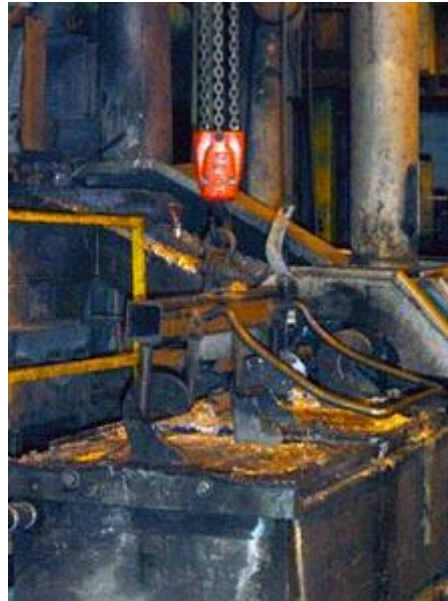
Lead tap at reverberatory furnace
