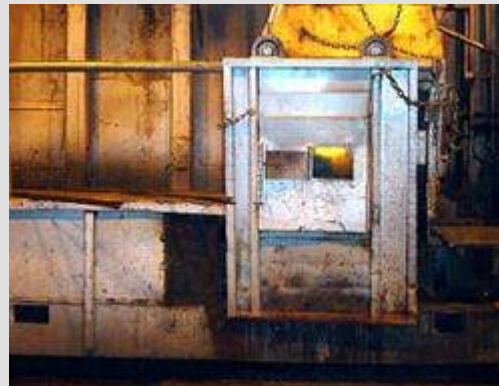
Reverberatory furnace tap hole hood
