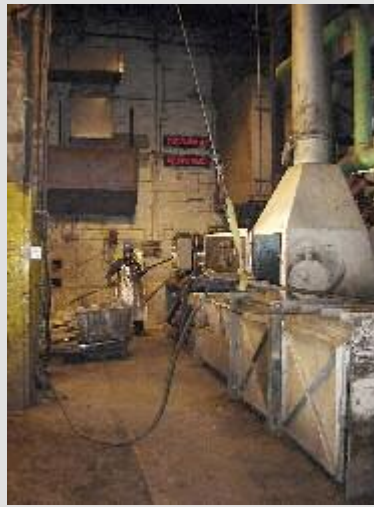
Slag side of blast furnace
