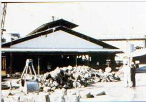
Fig. 5. Tetra ethyl lead (TEL) storage
