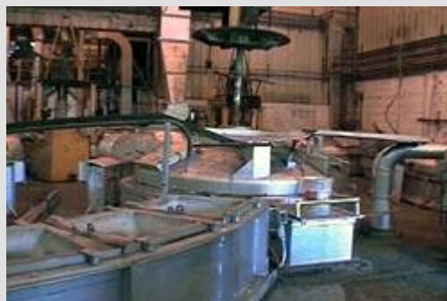
Fig. 1. Removing pump from enclosed refining kettle
