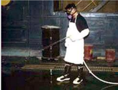
Fig. 2. Wetting surfaces to suppress dust generation
