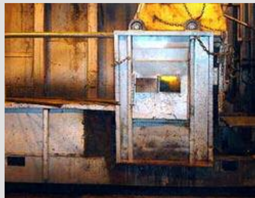
Reverberatory furnace tap hole hood
