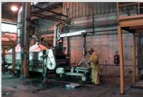
Fig. 4. Enclosed and exhaust ventilated star caster
