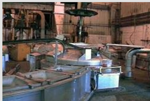
Fig. 1. Removing pump from enclosed refining kettle
