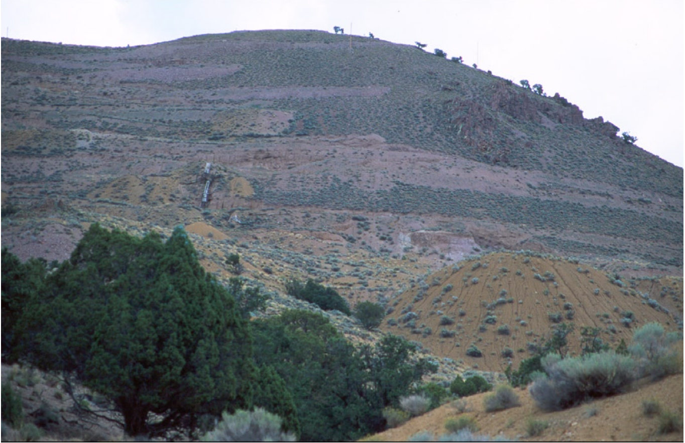
Figure 54. View of the area from which uranium was extracted, looking east toward Jungfrau Peak with goethite-coated waste-rock piles in foreground. The remains of an ore chute are visible just left of center near the site of an abandoned mine shaft.
