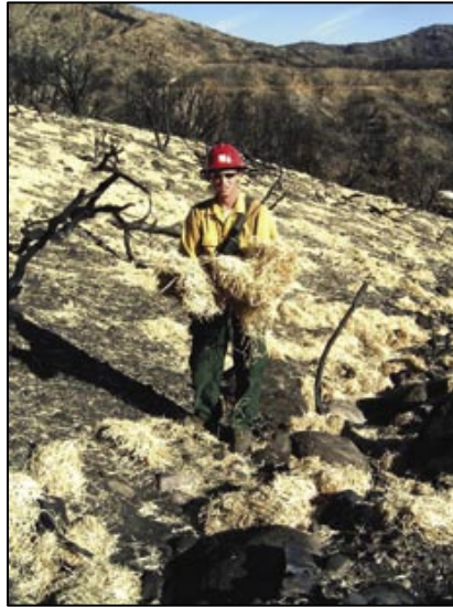
Figure 2.4. Hay, straw, and other crop residues being applied by hand (USDA/USFS, 2006).
