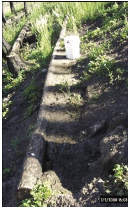
Figure 2.7. Downed logs are used in contour tree felling to trap transported sediment (USDA/USFS, 2006).
