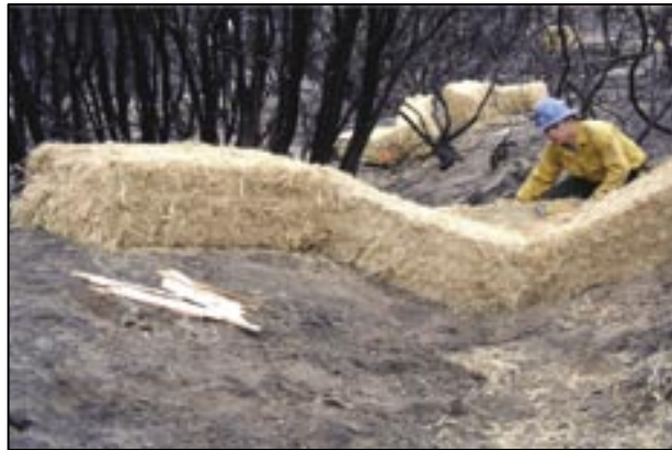
Figure 2.5. Straw bale check dams are installed in ephemeral or intermitting channels (UDSA/USFS, 2006).
