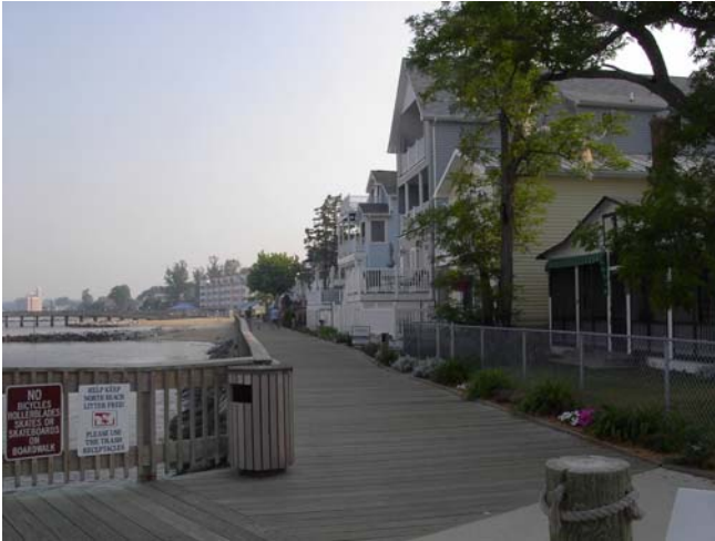
Figure 8.7 Public access along a bulkheaded shore. In North Beach, Maryland, one block of Atlantic Avenue is a walkway along Chesapeake Bay (May,2006).
