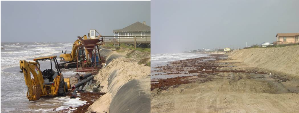
Figure 6.2 Geotube (a) before and (b) after being buried by beach sand at Bolivar Peninsula, Texas (May 2003).
