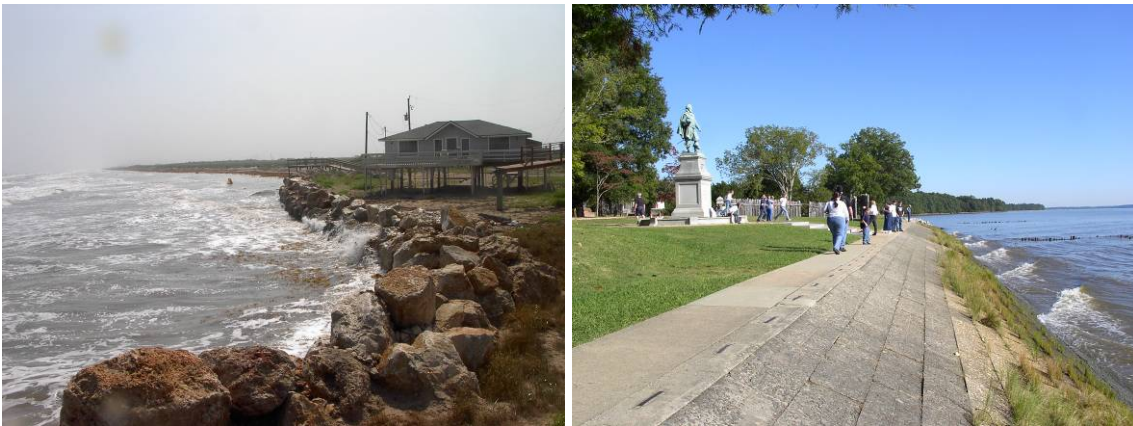
Figure 6.3 Two types of stone revetments (a) near Surfside, Texas and (b) at Jamestown, Virginia.
