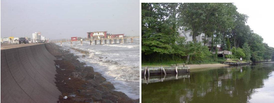
Figure 6.1 Seawalls and Bulkheads (a) Galveston Seawall in Texas (May 2003) and (b) Bulkheads with intervening beach along Magothy River in Anne Arundel County, Maryland (August 2005).
