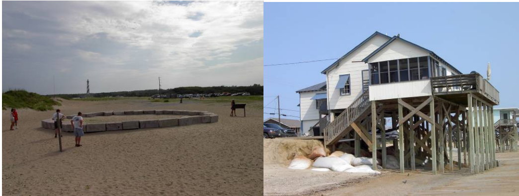
Figure 6.8 Relocating structures along the Outer Banks (a) Cape Hatteras Lighthouse after relocation at the Cape Hatteras National Seashore, Buxton, North Carolina (June 2002); the original location is outlined in the foreground, and.(b) a home threatened by shore erosion in Kitty Hawk, North Carolina (June 2002). The geotextile sand bags are used to protect the septic system.
