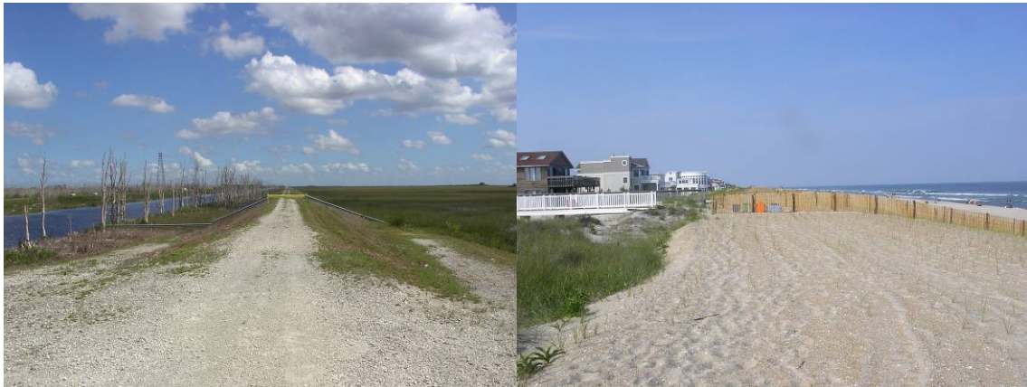
Figure 6.4 (a) A dike in Miami-Dade County, Florida, and (b) a newly-created dune in Surf City, New Jersey.
