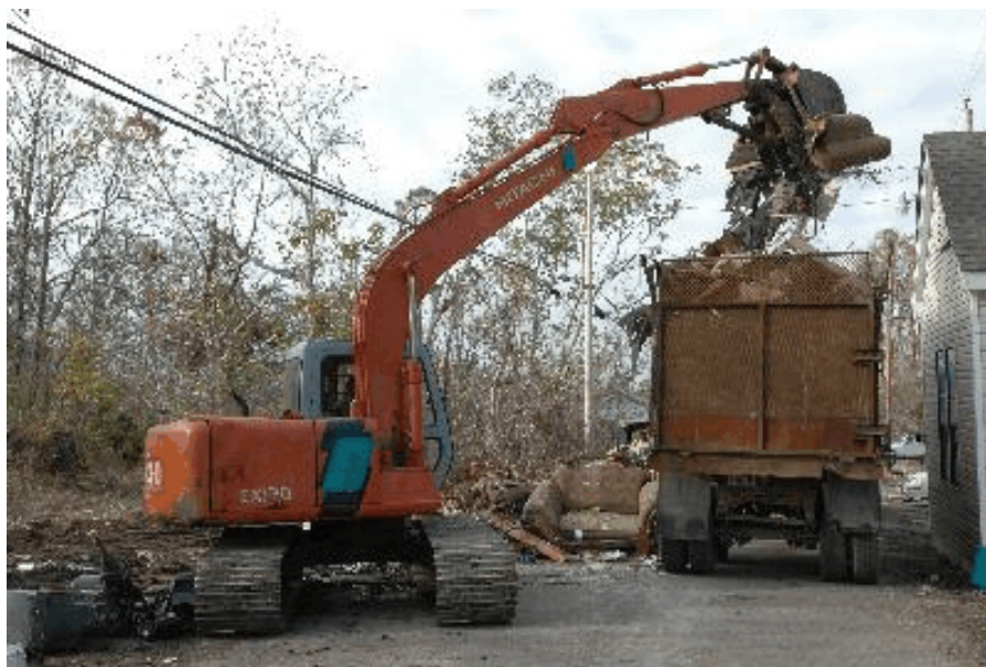
Figure 1 - Hydraulic Excavator Filling Debris-Removal Truck in Pass Christian, Mississippi
