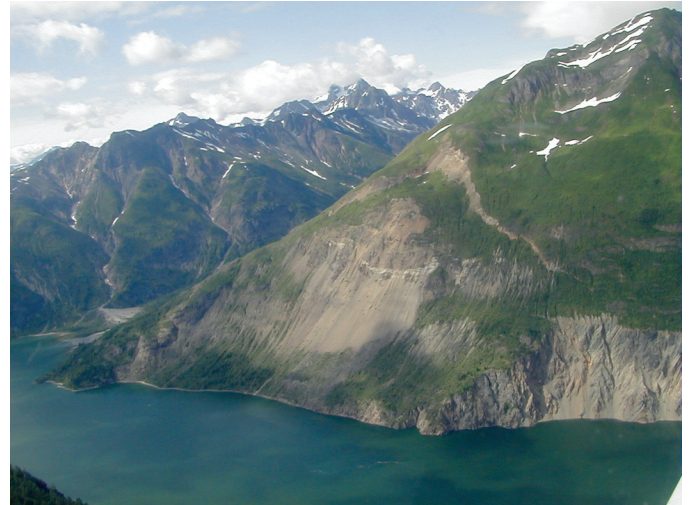
Figure 1. Detached landslide perched above the northern shore of Tidal Inlet, Glacier Bay National Park, Alaska. Photograph taken July 12, 2002.
