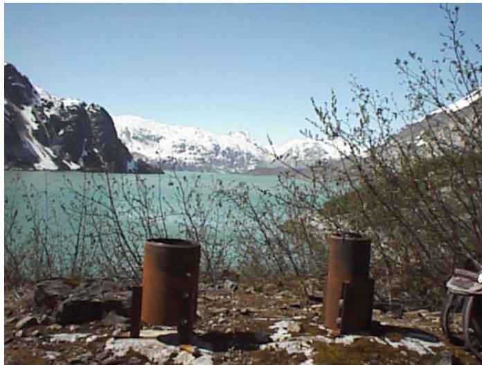
Figure 2. Typical monitoring set up at climate sites. Upper left photo shows white solar radiation shield housing temperature sensors and a tipping bucket rain gauge installed on 1-meter tall post at Muir Glacier. Photo on lower right shows the tipping bucket and electronic rain gauges in steel housings as mounted on the ground at the Riggs site. A post is only used where animals are unlikely to damage rain gauges, but preferred to reduce snow cover effects early in the winter season.
