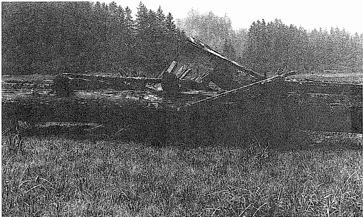
A fish trap on the beach at Excursion Inlet. The collapsed structure is the former watchman's shack.
