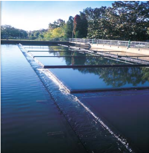
A sedimentation basin
