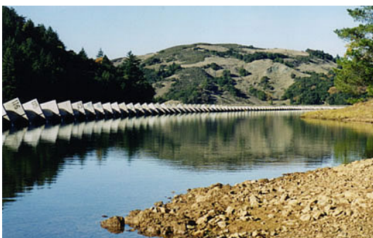
A reservoir and water supply pipeline
