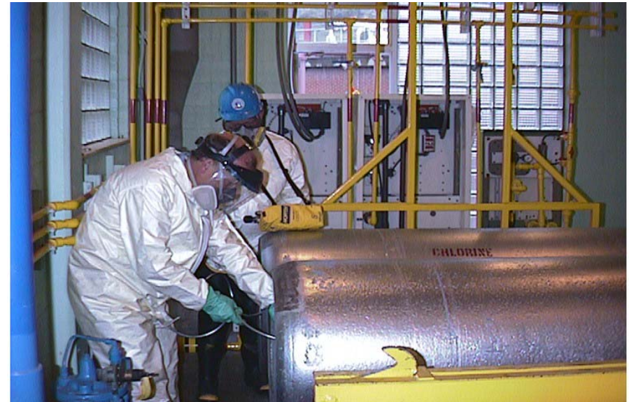
Workers in Montana changing a 1-ton chlorine gas cylinder
