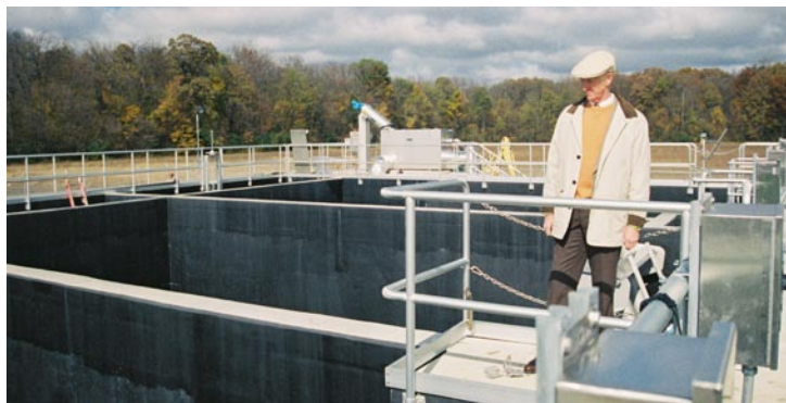
Mayor Fallows makes final inspections before the grand opening of a brand new wastewater treatment plant in Haskins, OH.
