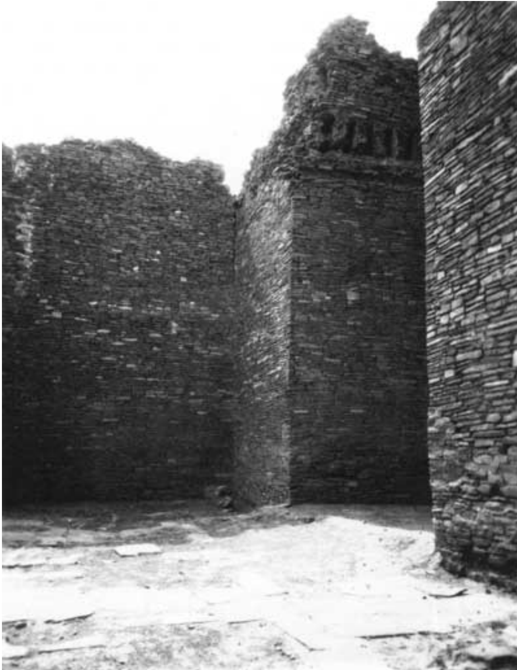
Figure 54. The west transept and apse of the church of Quarai in the fall of 1937. In the northeast corner of the transept the west side altar base still stands, and closer the last traces of the main altar stairs remain at the west side of the apse. The socket for the stair bannister on the corner of the apse has been filled. In the foreground at the lower right corner of the picture, the top of the east side altar base is just visible. The surviving flagstone of the transept can be seen, and the rectangular areas of bare dirt in front of each of the altars. High on the west wall of the transept, patches of white wall plaster can be seen. Some of this patch still survives today. High in the apse the horizontal socket of the retablo support beam runs beneath the sockets of the apse roof vigas. Above these, the severe collapse around the sockets of the transept roof beams is visible. This collapse was caused by the burning out of the main viga that ran across the north face of the transept just under the corbels of the transept vigas. It supported
