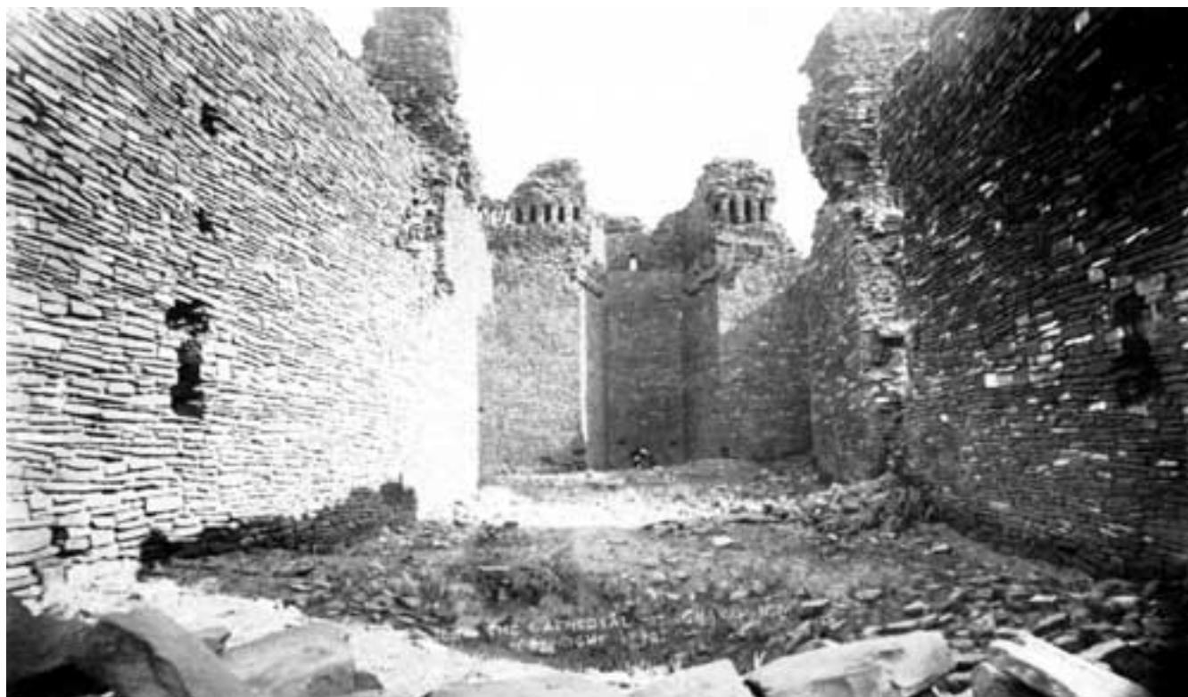
Figure 36. The interior of the church of Quarai in 1890. This is the earliest detailed view of the interior wall surfaces of the church. A number of important details can be made out. In the north wall of the apse, the hole chopped through the wall by treasure hunters is easily visible. To the left and right of this hole on the apse wall are the sockets for the lower supports for the retablo. At the left and right corners at the mouth of the apse can be seen the sockets for the bannisters of the stairs of the main altar. On the left wall of the nave, the collapsed stonework above the lintel of the west window can be seen, as well as the neat masonry that sealed the window in colonial times. The stonework fell in above the window because the lintel woodwork burned out all the way through the wall during the fire in ca. 1830. Closer to the camera on the left can be seen the multiple sockets of the choir loft. The lowest socket is a three-part outline for the cobel beneath the main viga, the viga itself, and the lower railing of the choir loft bannister above. Above this triple socket, and a few inches north, are the middle and upper sockets of the choir loft bannister. On the right, or east wall, of the nave, an identical set of sockets can be made out. Closer to the transept, the notch of the east window of the nave can be seen. The sill of the window has collapsed almost to the level of the fill within the church. The fill at this time is only about three feet deep. Photograph by Charles Lummis, 1890.
