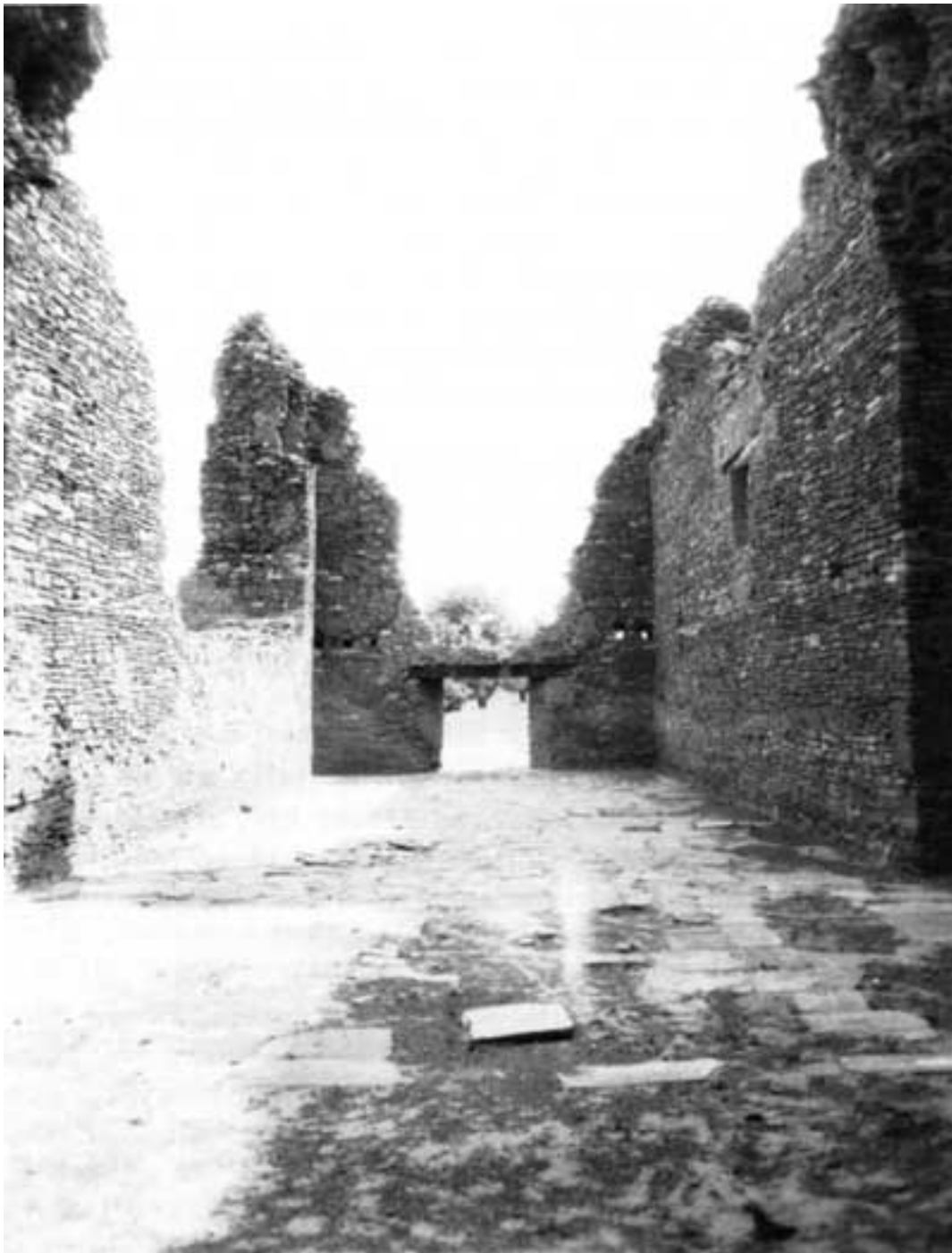
Figure 60. The nave of the church of Quarai in the fall of 1937. The photograph was taken after the completion of the first excavation and stabilization of the building. All of the surviving flagstones of the church floor remain undisturbed.
