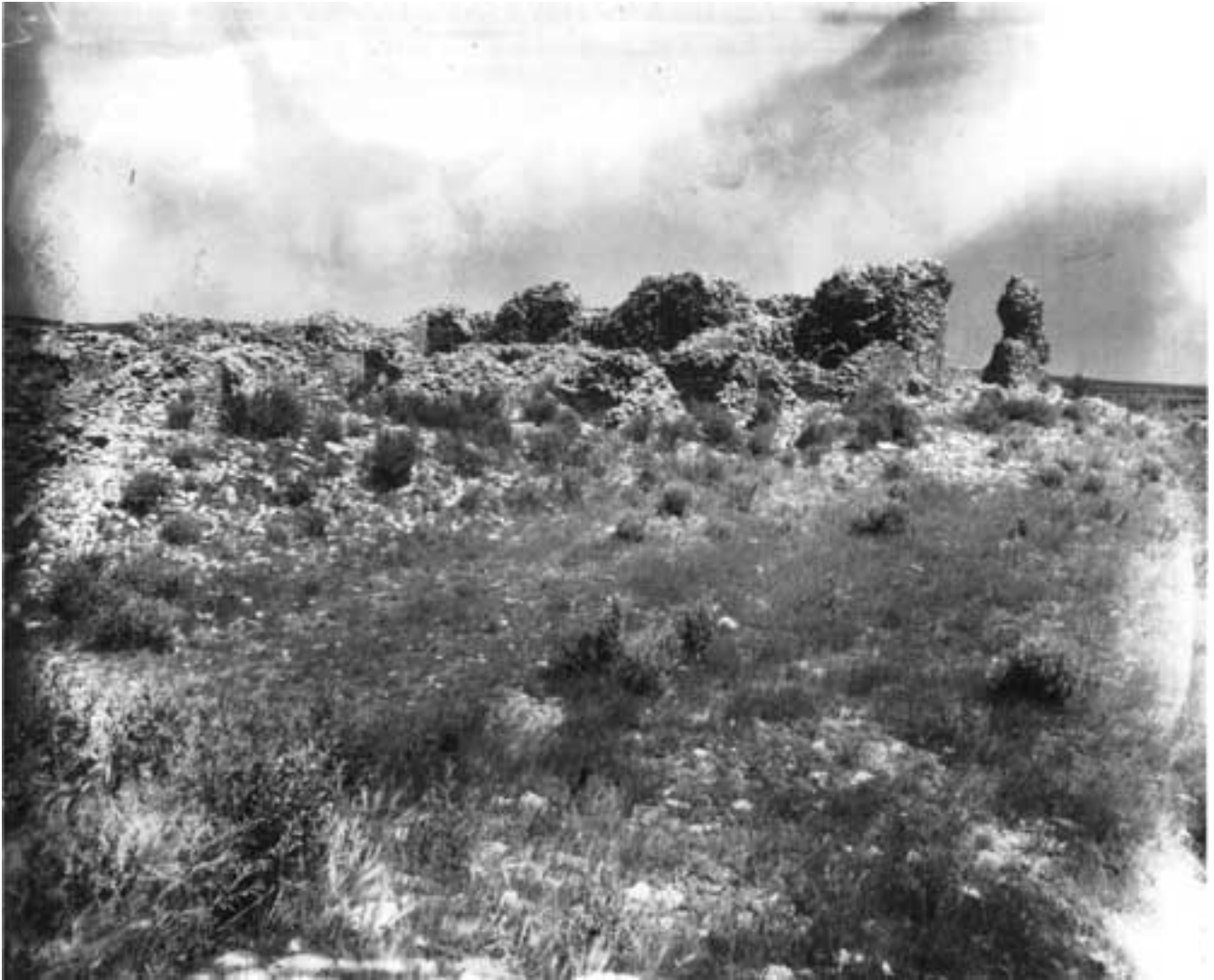
Figure 56. San Buenaventura about 1920, taken from almost the same spot as Bandelier's photograph in 1883. The tremendous loss of wall fabric through the theft or, in a few cases, the decay of lintels, is obvious.
