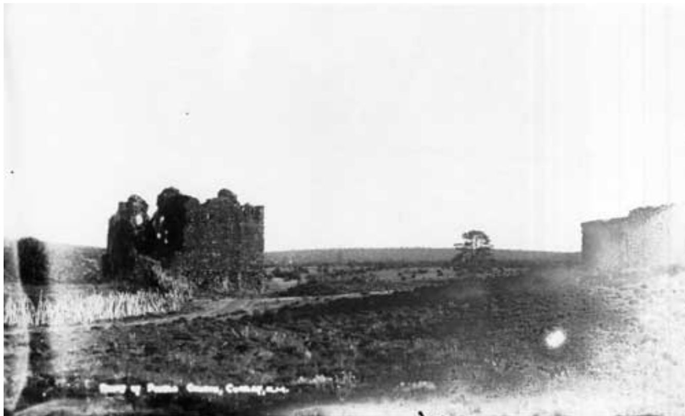
Figure 35. Quarai from the north in 1890. Lummis was the first photographer to record the details of this side of the church. At the right edge of the picture, the North House still stands to its full height. On the left corner of the church the walls of room 6 still stand to the top of the second story, and one roof viga remains in place against the north wall of the east transept. The notch of a window at the second floor level can be seen in the north wall of the room. At the top of the apse, the ventilation opening can clearly be seen, as well as the notch in the top of the wall where the canal that drained the apse roof had penetrated. The road to Abó from Punta de Agua curves around the church with a jacal fence along its east side. The road and fence were both recorded by Bandelier on his plan of the pueblo and mission made from the notes and sketches of his 1882 visit.
