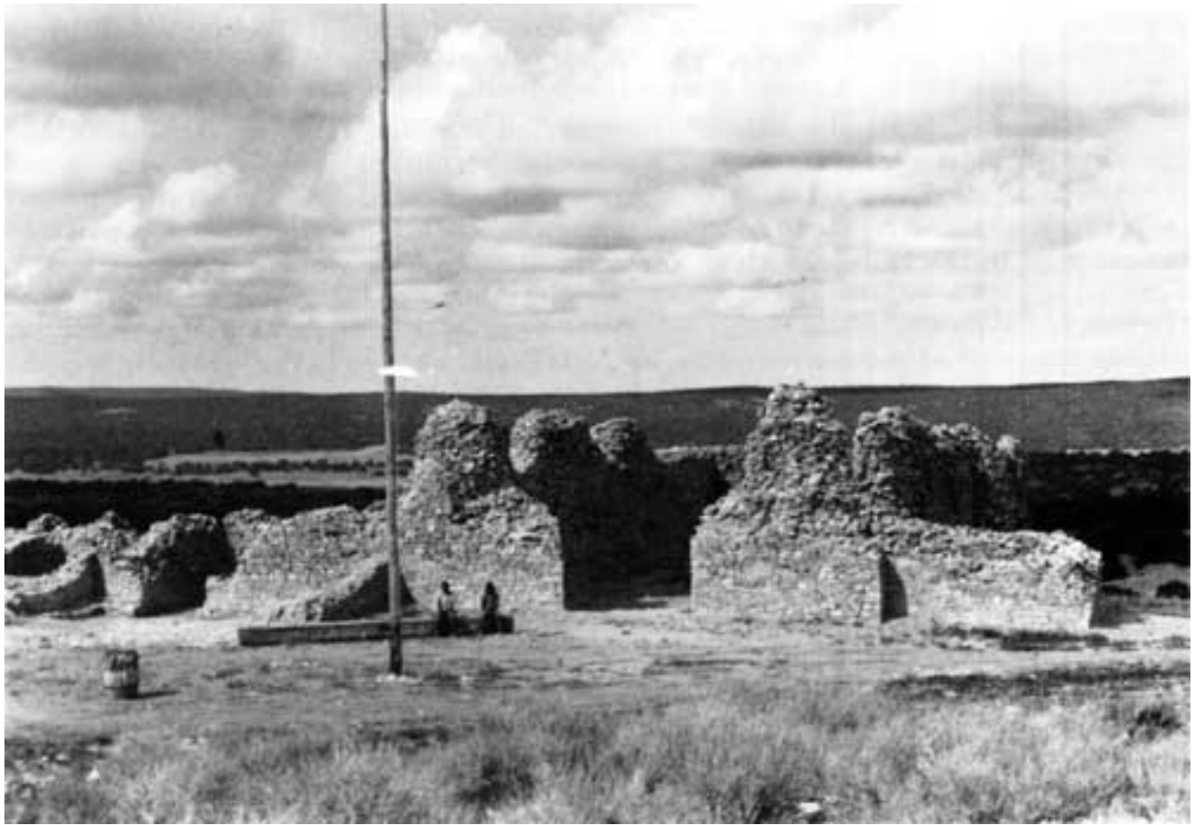
Figure 63. San Buenaventura in the 1940s. The lintel beam has been returned to the site, and is on the ground behind the flagstaff with two people sitting on it.
