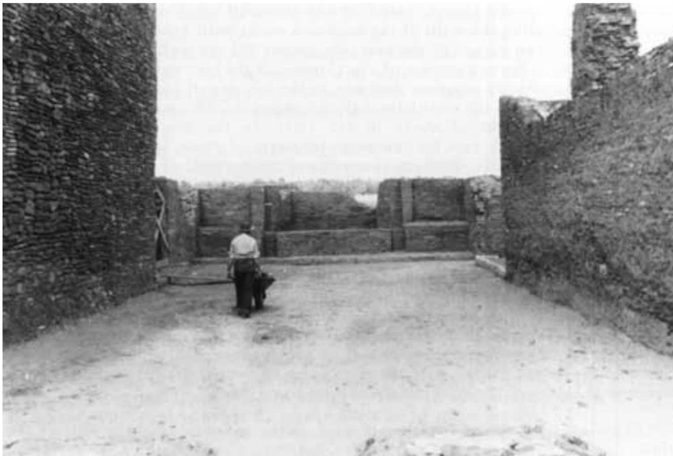
Figure 58. Abó in 1939. The interior of the church in the final stages of cleanup and stabilization. Replacement beams have been cut and set into the floor along the edges of the side chapel altar platforms and in front of the main altars. Stabilization of the side walls of the sanctuary near the side altars has not yet been carried out.
