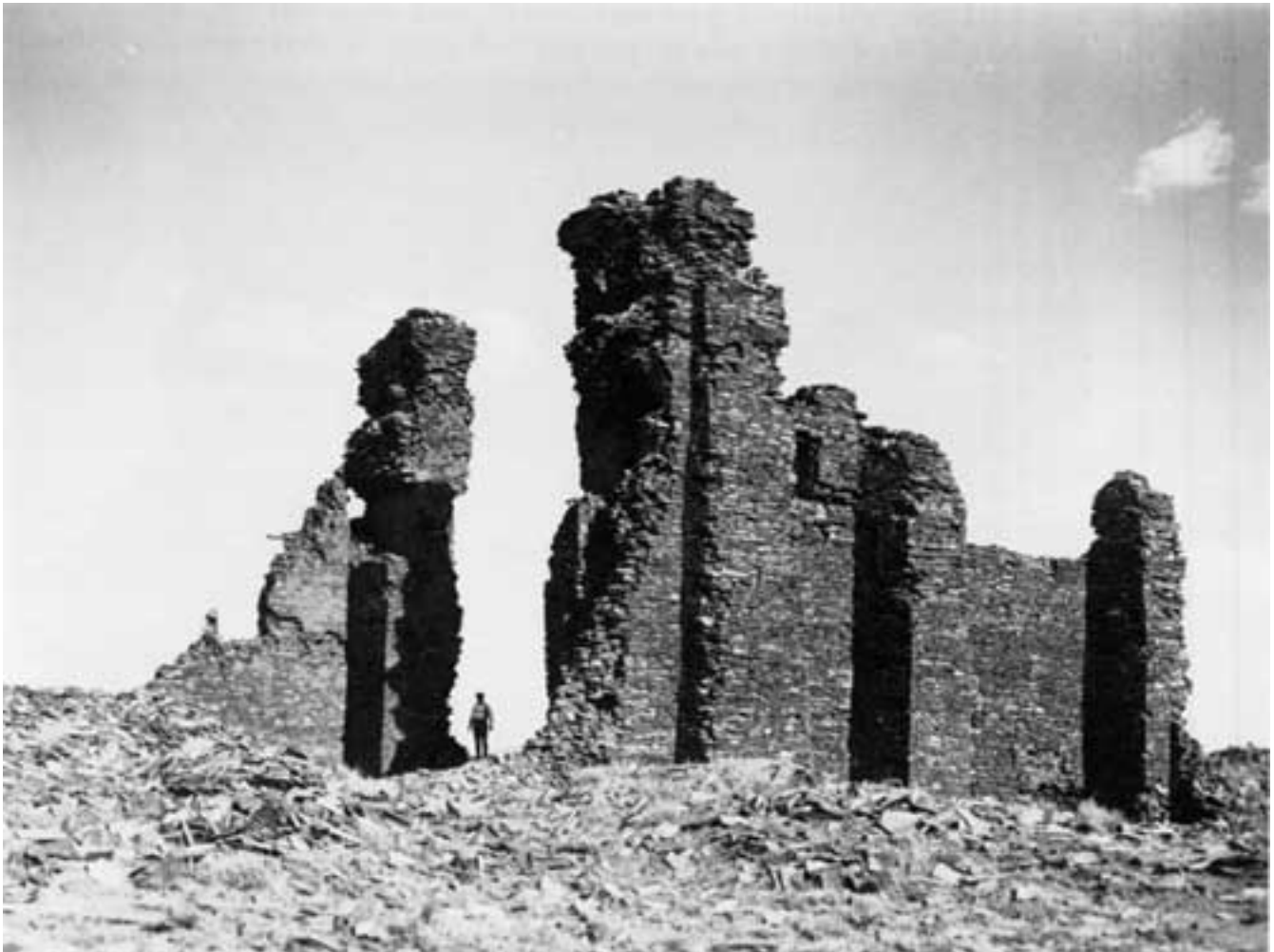
Figure 28. Abó from the northwest in 1916, by Jesse L. Nusbaum. The walls of the sanctuary and side chapels have fallen, except for the buttressed area of the bell tower, and the tower buttress on the east side. The southernmost bottom corner of the balcony doorway is visible just to the right of the figure sitting on the sill of the doorway on the wall. Below the doorway can be seen the irregular traces of the sockets for the eastern balcony. On the shadowed north face of the east tower buttress, the dark patches of the socket for the viga that supported the balcony can be seen, with the sockets of the balcony railing above it. The large depression in the wall above the railing sockets is the socket for the east end of the lower clerestory vigas and corbels; the hole through the wall at this point marks the end of the vigas themselves where they penetrated to within inches of the outer surface of the wall. Several feet above this is the smaller indentation of the upper clerestory viga socket, and in the irregular wall surface above this and below the crenelations are the sockets of the vigas and corbels for the high roof above the clerestory. A similar series of sockets can be seen in the bell tower section of the west wall, closer to the camera.
