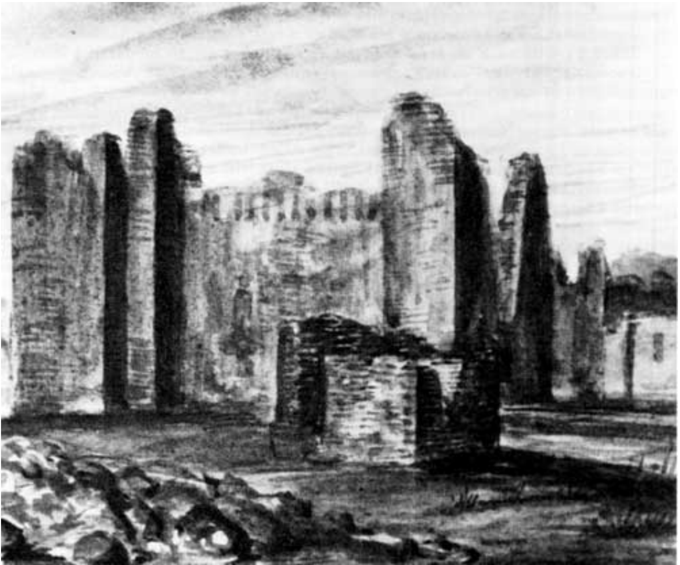
Figure 32. Quarai as painted by James Abert on Wednesday, November 4, 1846. In the foreground is the ruin of Mound J House, with the notch of a collapsed window on the right, or south side. Immediately behind it is the baptistry of the church. Abert indicates that he could see the sockets for the roof vigas of the nave from the outside of the building, meaning that the stonework between the sockets still stood to the height of the tops of the beams in 1846. To the right of the facade of the church, the choir loft stairwell and belltower still stand to the height of the top of the second story window. Just to the right of the belltower rooms is the gap where the portería has fallen in, and then the facade of the convento with a window opening, probably into the east hall. The rooms added on the southeast by the Luceros are out of sight to the right.
