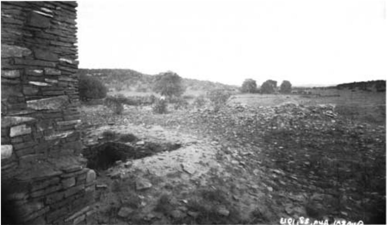
Figure 51. The area of the sacristy of Quarai in 1913. Lummis stood on top of the stub of the wall of room 6 to take this photograph. Just past the corner of the transept, the hole excavated into the sacristy can be seen. In the middle ground the walls of rooms 11, 12, and 13 have all fallen to heights of about one or two feet on the side toward the camera. On the east side, the walls stand four or five feet above the sloping rubble.
