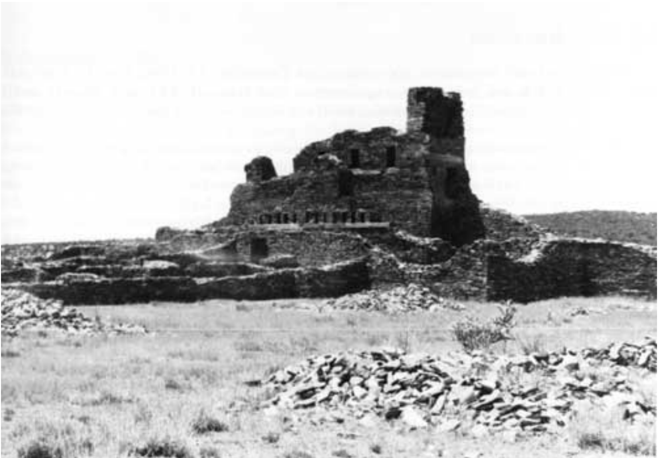
Figure 59. Abó as it appears today. The bell tower area is about 5 feet lower in this picture than in the previous photographs, but its top has been reconstructed to have the same general appearance as it had before the removal of the upper masonry. This demolition and remodelling occurred in 1972. The lower four viga stubs set in the north face of the tower by Toulouse are still in place, as are the viga sections in the east face of the west wall and under the sacristy roofbeam sockets, but the upper pair of viga stubs in the tower are gone, removed in 1958. The wall for the first four feet above the surviving viga stubs is refaced, the result of the work of 1972.
