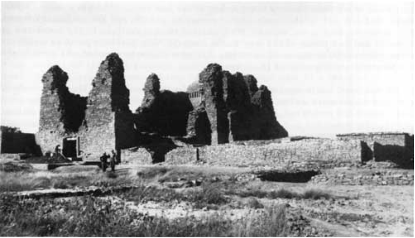
Figure 61. Quarai during the stabilization by Wesley Hurt, October, 1939. At this date the terrace in front of the church had been restored and the north wall of the west transept stabilized and built up to the height of the adjoining tower. The scaffolding has been moved into the apse. One strut of the scaffold is visible at the left edge of the tower at the south side of the east transept. Courtesy Museum of New Mexico, # 6666.
