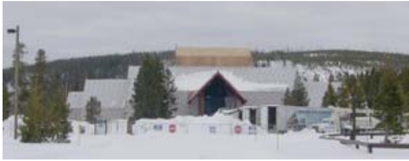
The new Old Faithful Visitor Education Center will be completed in 2010. It is being built to meet "Gold LEED Certification" (see previous page).
