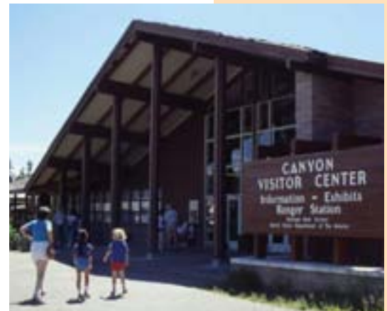
This Mission 66 era visitor center was renovated and remodeled into the Canyon Visitor and Education Center, which opened in 2006.
